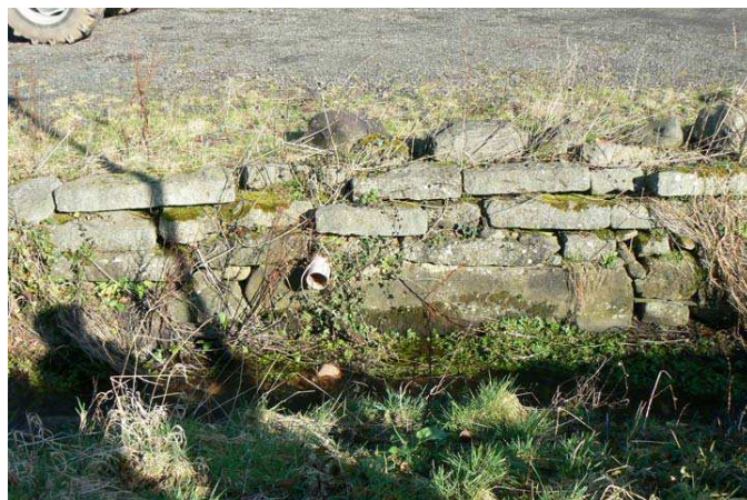
Low stone built retaining wall to sides of burn
