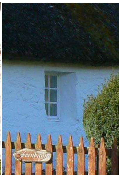
Small window opening, with frame set deep into the thick walls
