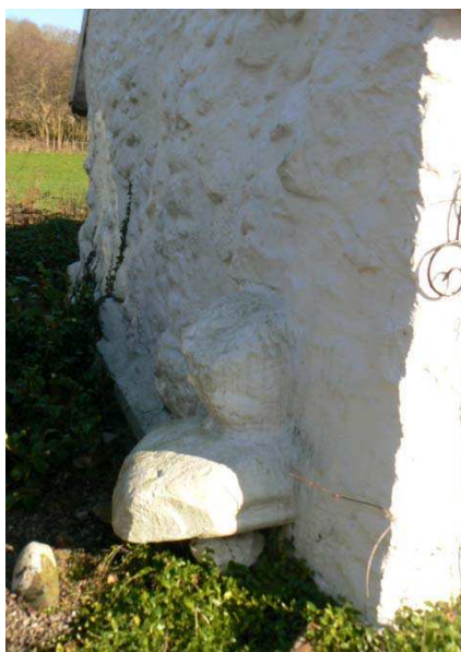
Picture shows slightly tapered walls and projecting stones
