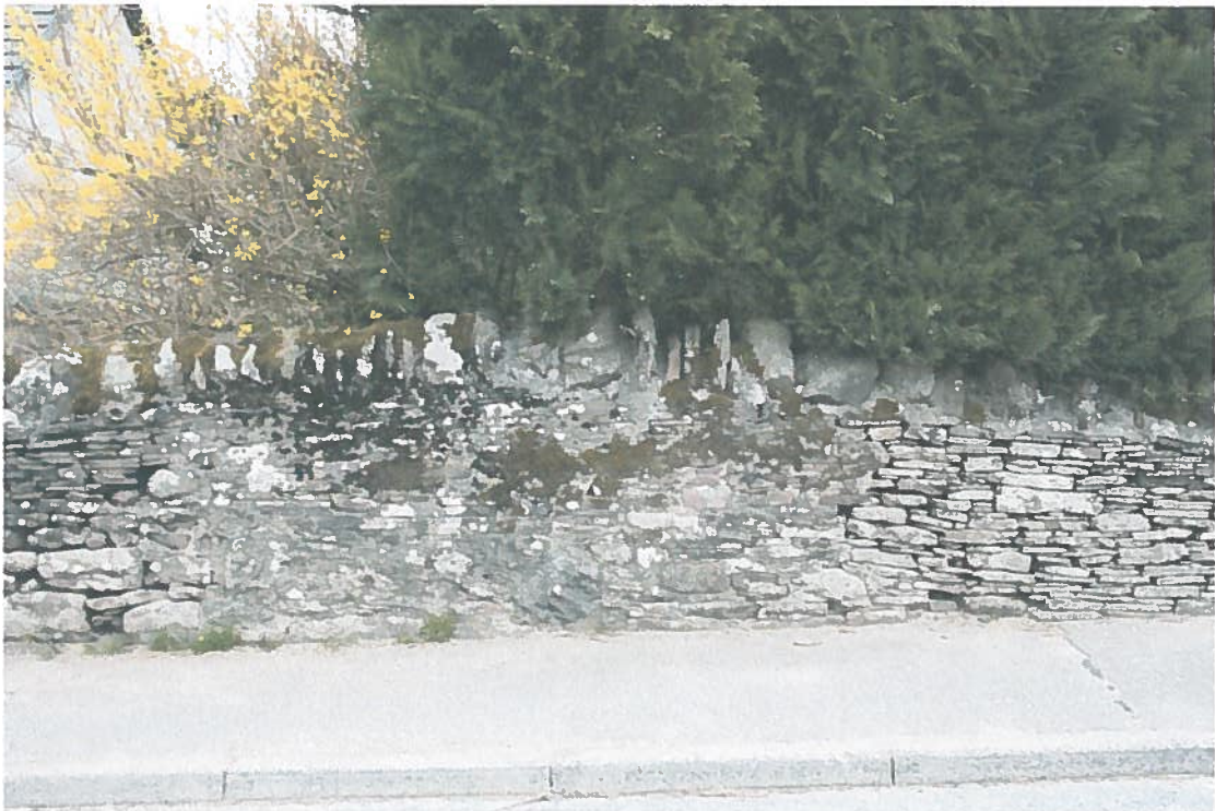
Picture 4 Stonewall at mid-point of Castleton Road showing poor condition and heave due to tree roots
