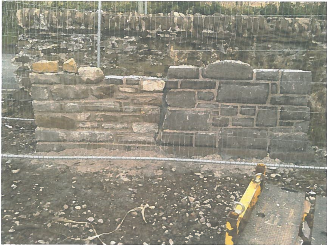
Picture 11 showing stone samples - weathered yellow sandstone on left and grey sandstone on right, with existing stone wall behind
