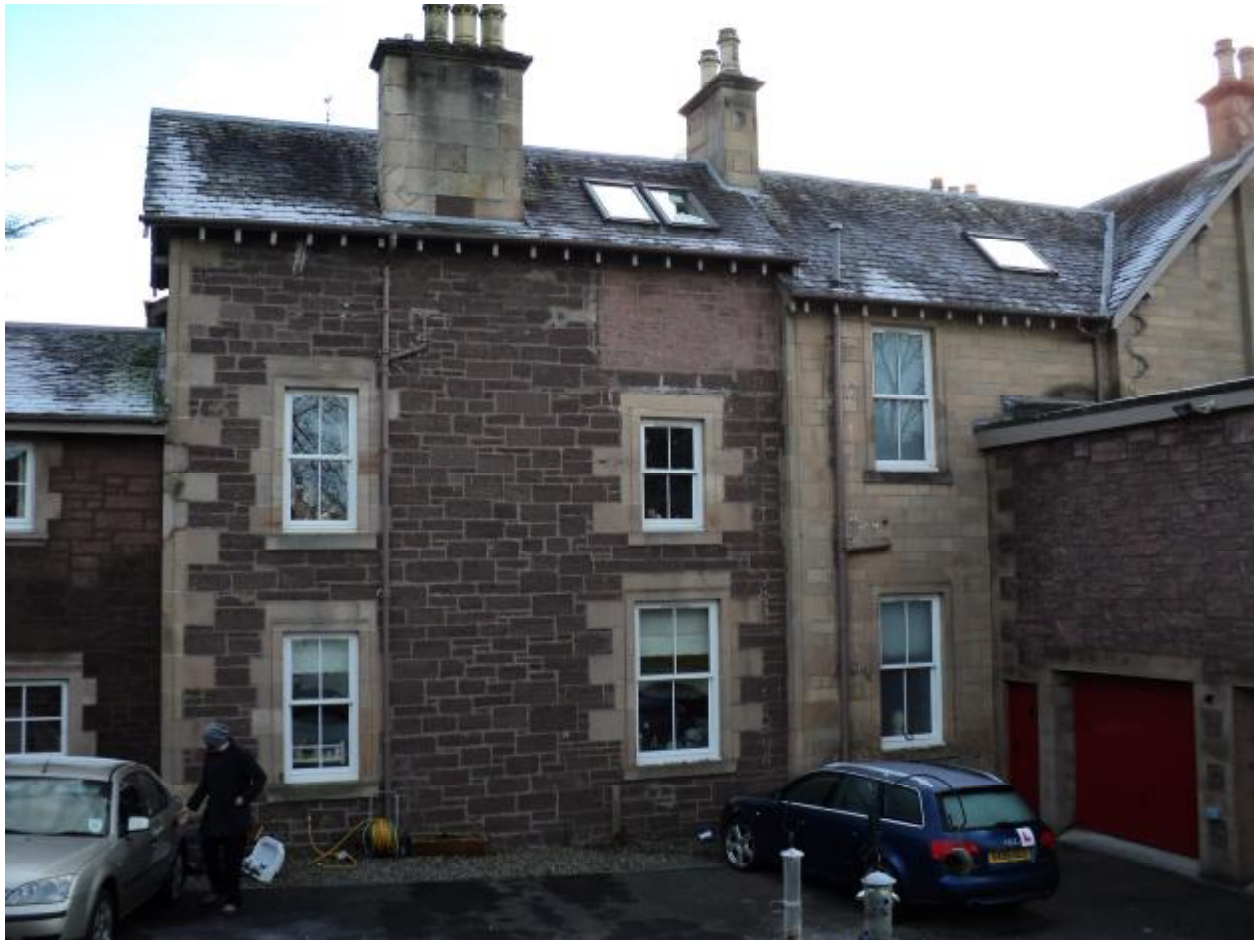
KNOX HOUSE – PHOTOGRAPH OF EXISTING PERTSHIRE SANDSTONE WALLING TO NORTH ELEVATION
