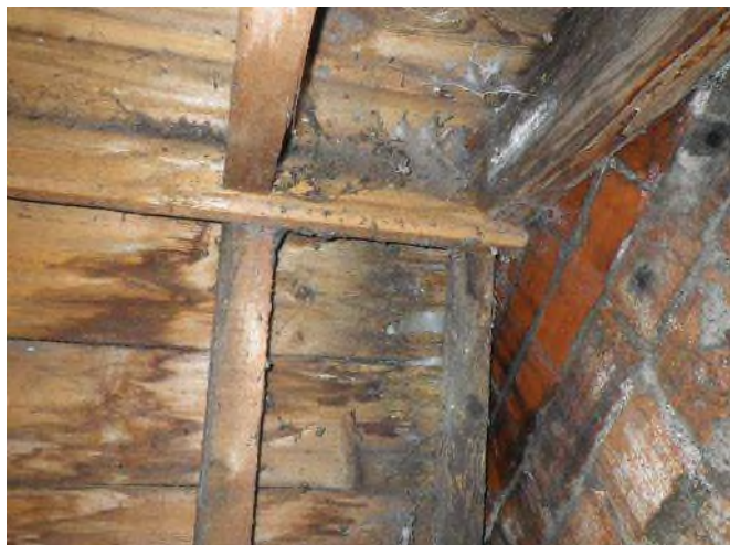
Photo 9: Gaps and staining at east end of building allowing access by bats
