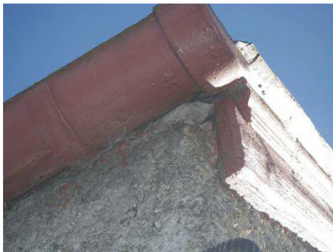
Photo 4: Deterioration at corner of building between wall and barge board
