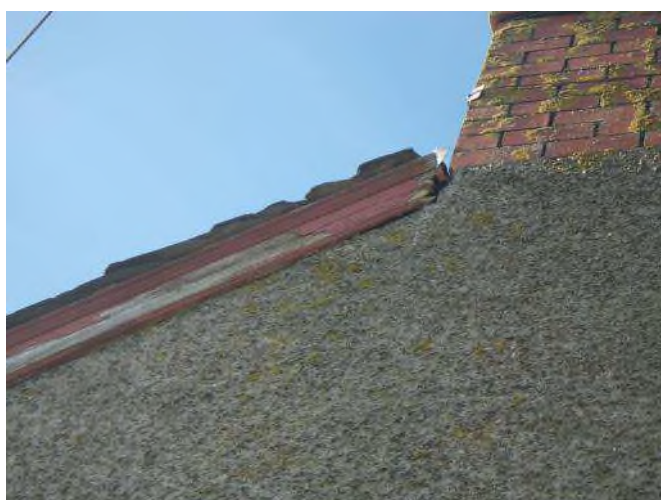
Photo 3: Deteriorated barge board at chimney
