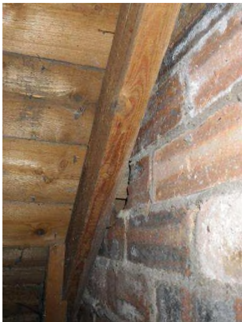
Photo 9: Gaps and staining at east end of building allowing access by bats
