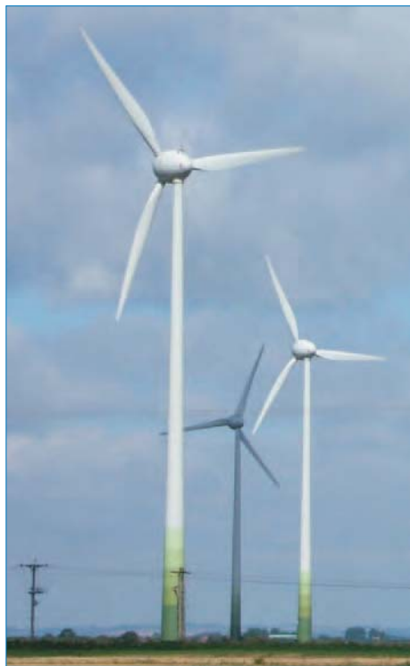
Alternative wind turbine proportion – these images show the contrast between blade length and tower height, which affects the overall visual range.
