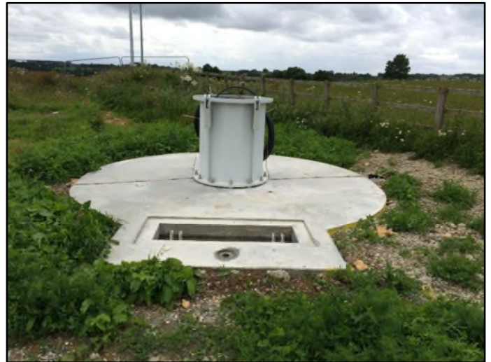
Diagram 4: A typical H15 Foundation
