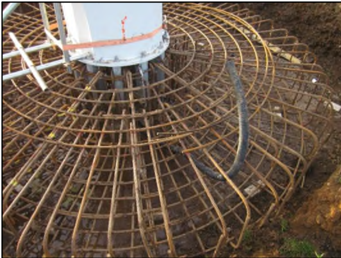
Diagram 3: Example of re-bar cage installed onsite
