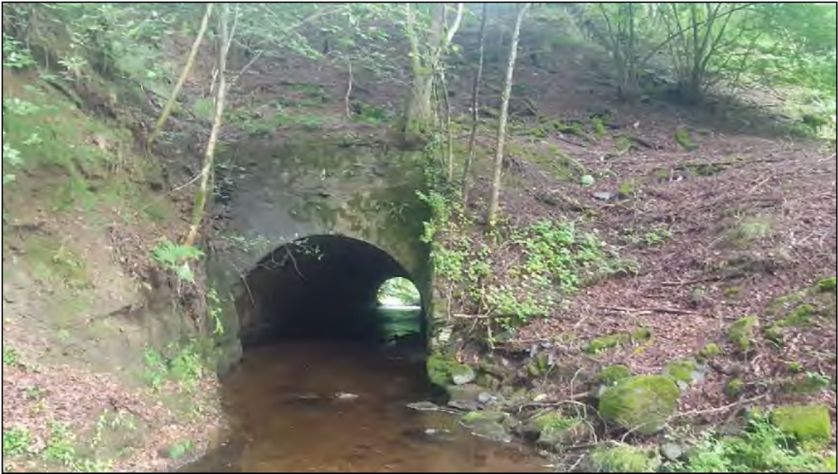
Photograph 21 - Looking east (downstream) to the entrance to the large arched culvert under the A823 road embankment.
