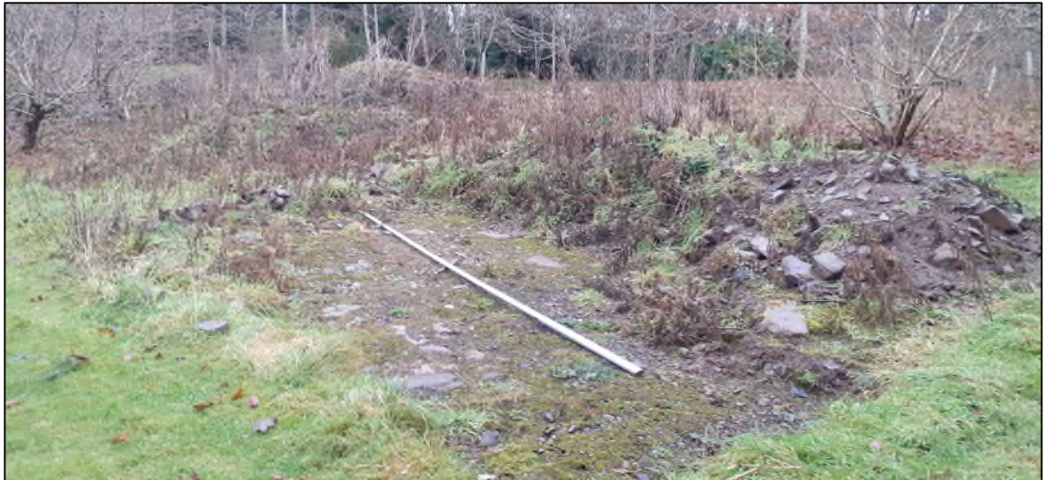
Photograph 1 - Looking north over location of survey points 1 and 2 (roughly at either end of the surveying staff lying in the excavated area. Note the exposed foundation stones in the stripped back area, original garden ground in foreground to left and right, and mounds of demolition rubble behind.
