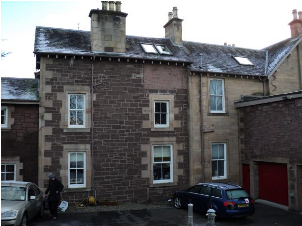
KNOX HOUSE – PHOTOGRAPH OF EXISTING PERTHSHIRE SANDSTONE WALLING TO NORTH ELEVATION
