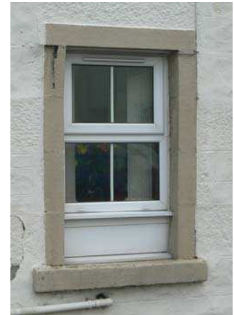
Example of an inappropriate window replacement
