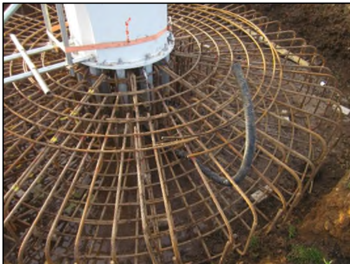
Diagram 3: Example of re-bar cage installed onsite
