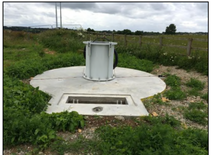
Diagram 4: A typical H15 Foundation
