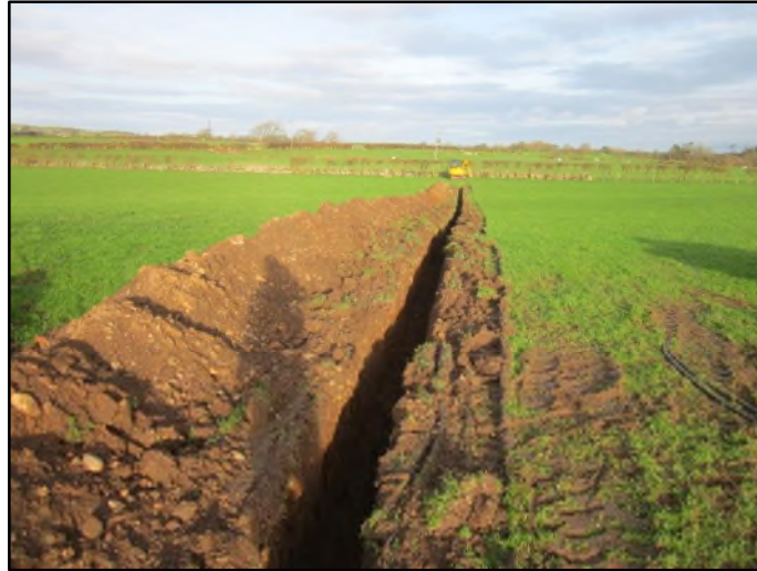
Diagram 5: A typical trench for laying of the cable
