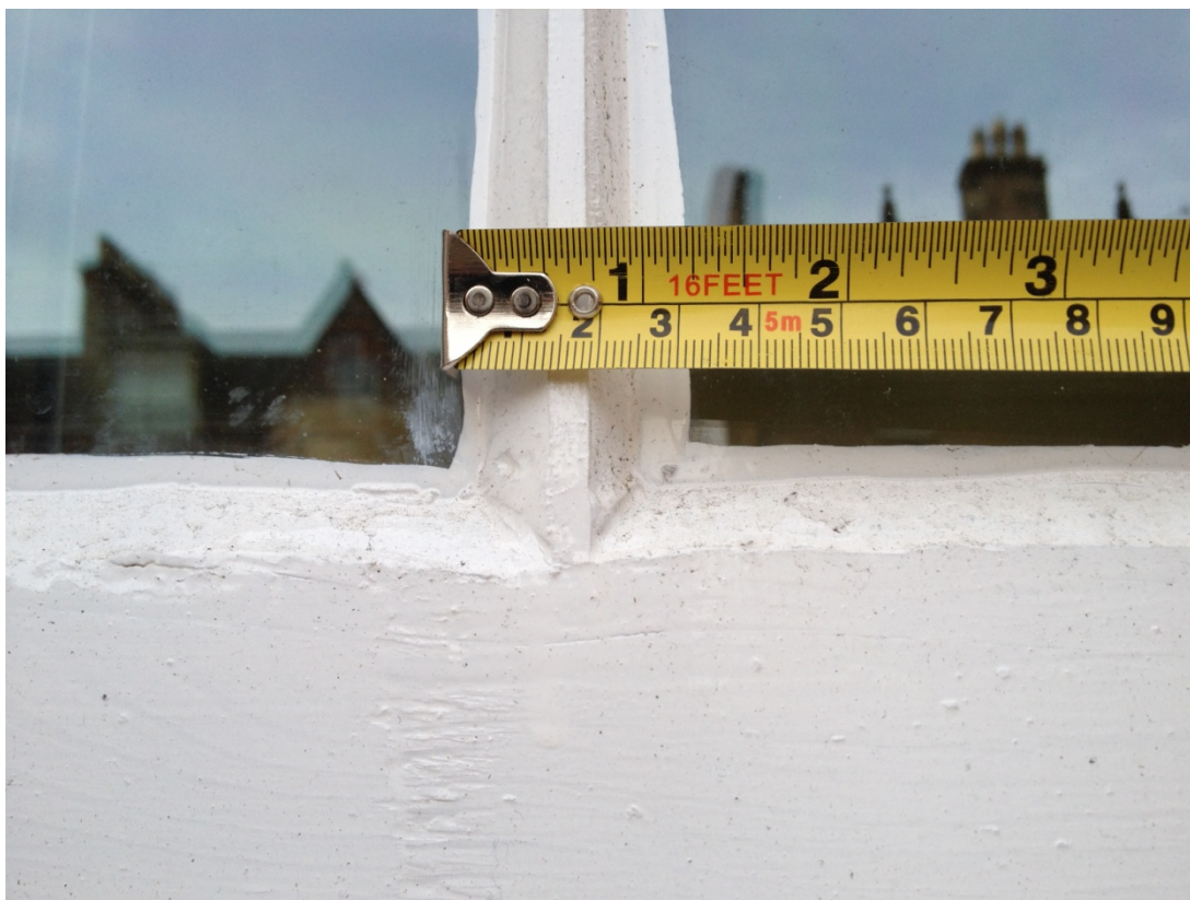
Astragal of Criagie primary school double glazed window: 23mm wide. Paint gives appearance of 37mm wide.
