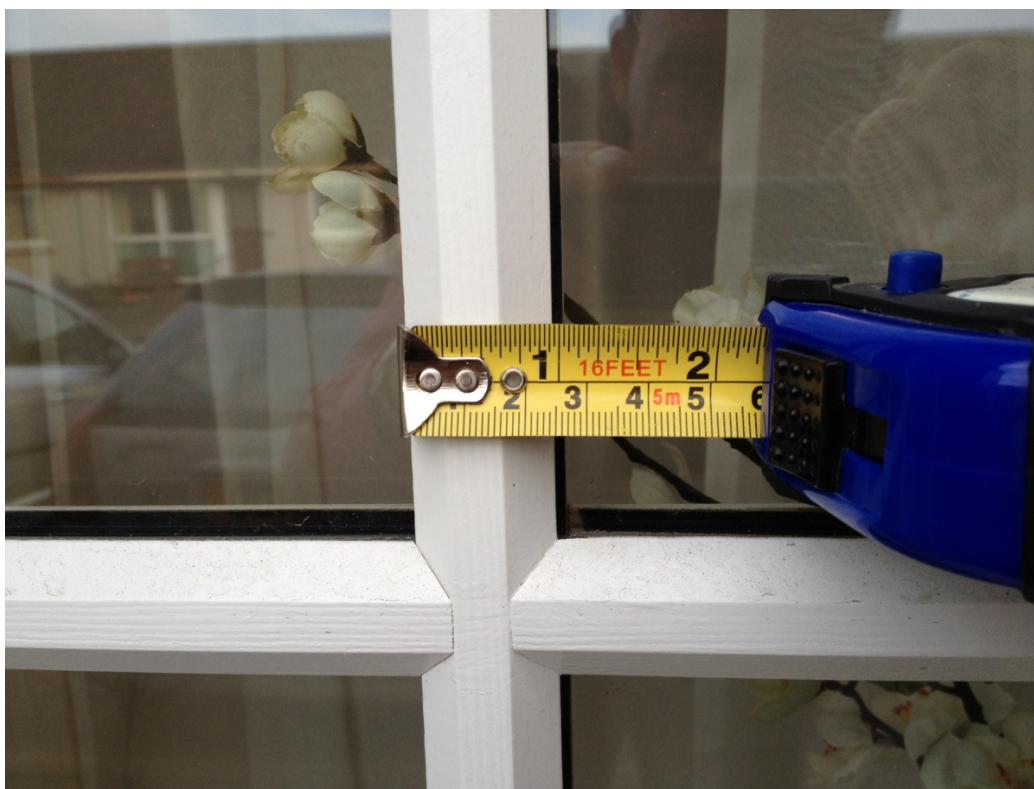
Pitheavlis new wooden sash & case double glazed windows, astragal 24mm wide. Appearance 24mm. Windows match those upstairs. No difference in appearance from roadside.
