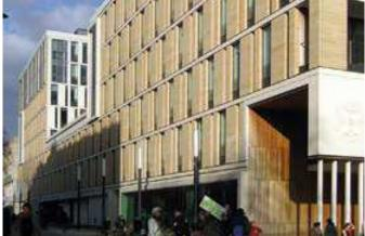
**Informatics Forum – Charles Street** Sandstone is built into vertically proportioned panels which are used to order the design of the elevations.
