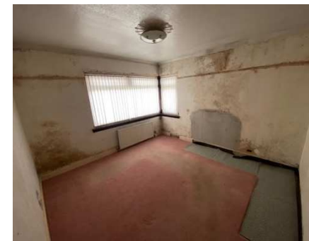
Figure 1: showing the damp in the existing house (main bedroom)
