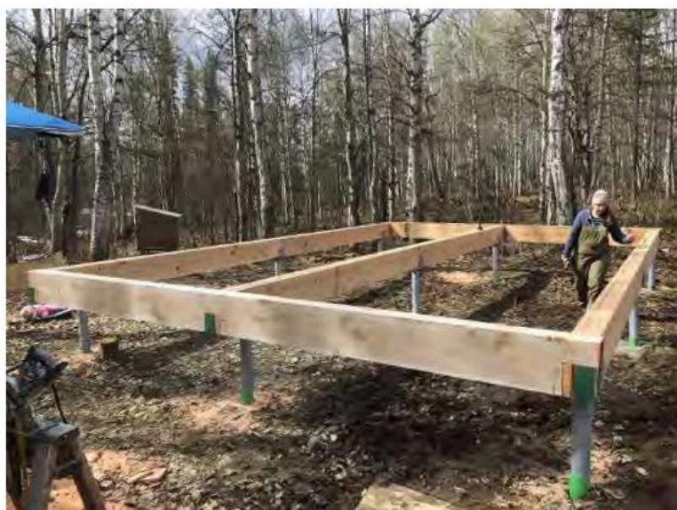
▲ Photo showing screw piling in close proximity to existing trees
