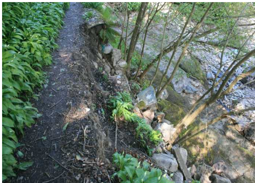
Plate VII - Wall collapse in the vicinity of the 2012 Landslip (Photo dated Dec 12)
