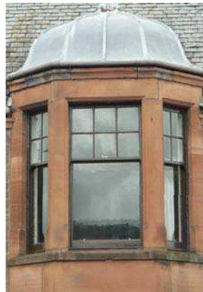
Unusual historic Crittal steel window (middle). Original sash and case window with historic glass (right).
