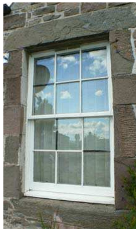
Examples of poor replacement windows in historic buildings, including failed plant-on astragals (right).
