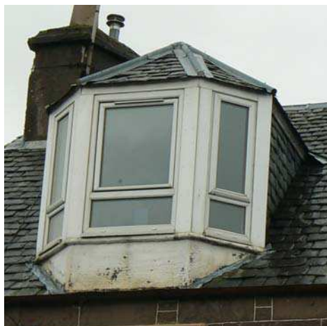
Examples of poor replacement windows in historic buildings, including failed plant-on astragals (right).
