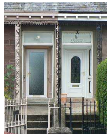
Poor replacement doors, not coherent with character of building (left)
