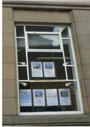
Unusual historic Crittal steel window (middle). Original sash and case window with historic glass (right).
