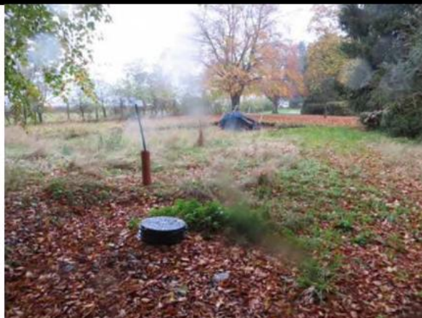
View towards SW, across application site, towards path running to the W of the site. (Excavated foundation of pool house and installed services in view).
