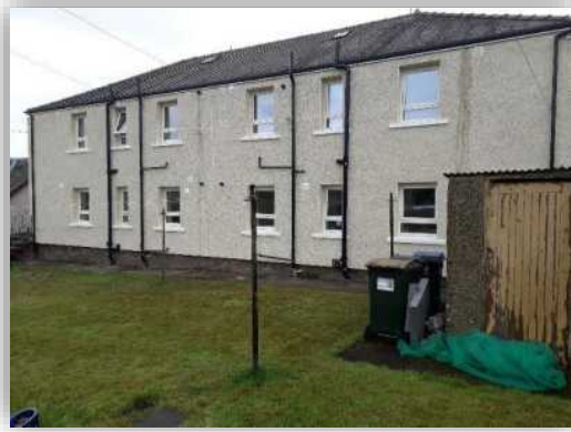
External Wall Insulation - High Street, Alyth
