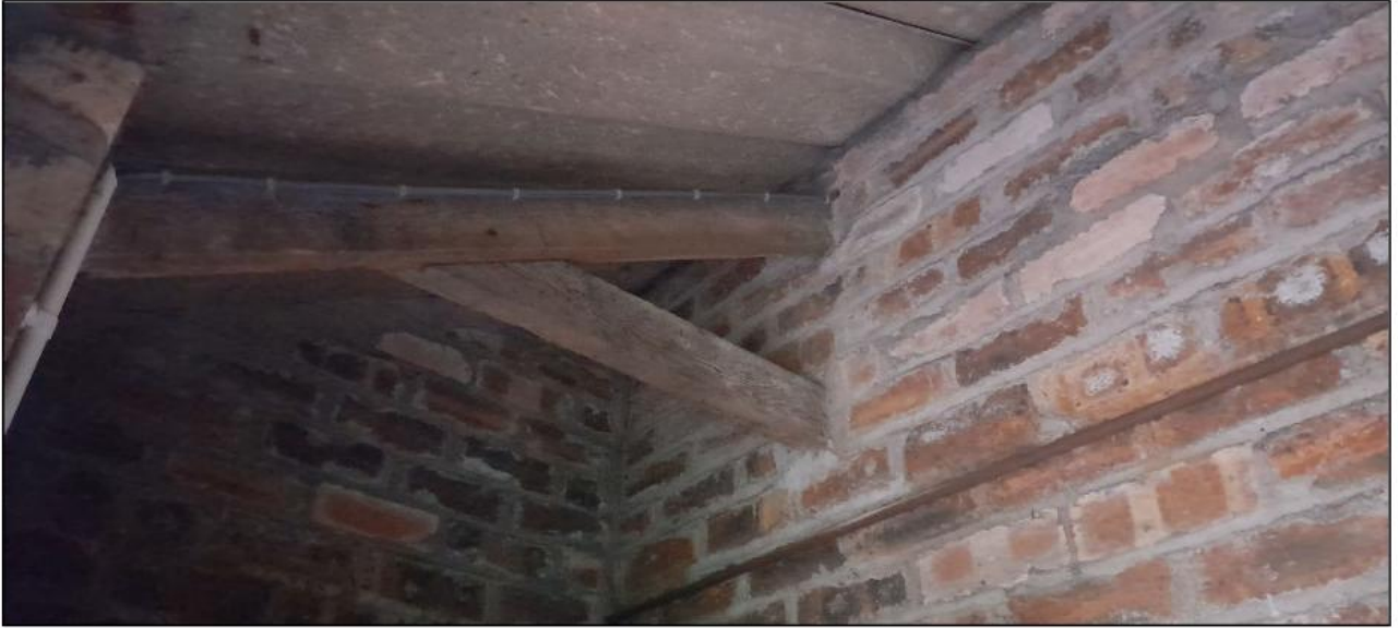
Photo 3: Inside the storage space
