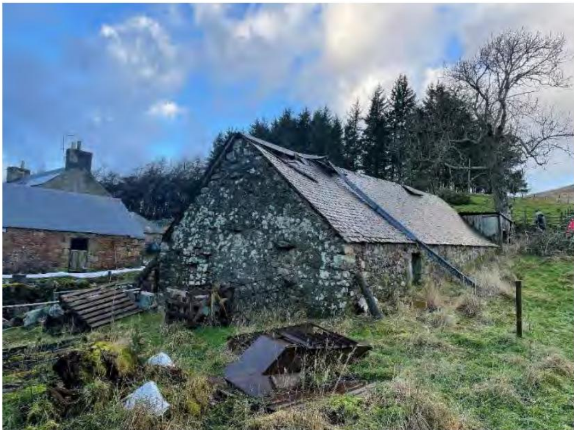
Figure 7: Picture of the steading showing current disrepair
