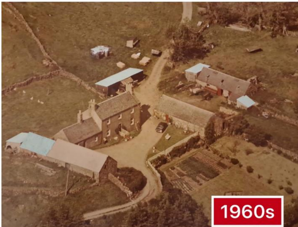
Figure 6: Former lean-to located to north and south of steadings. Shown by tin roof
