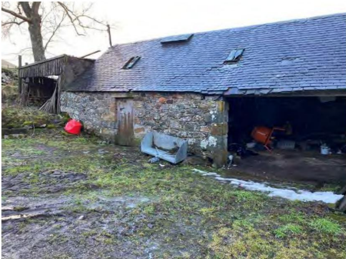
Figure 8: Picture of the steading showing current disrepair
