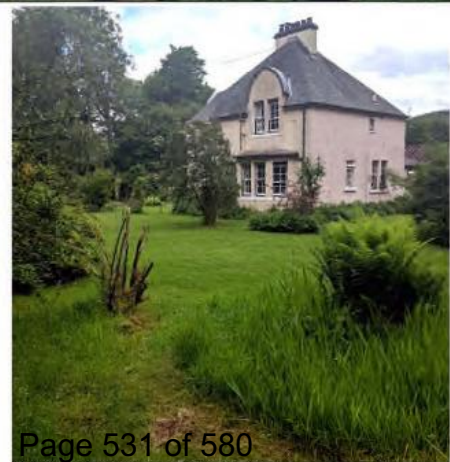
V02 - View of house from SE corner of garden
