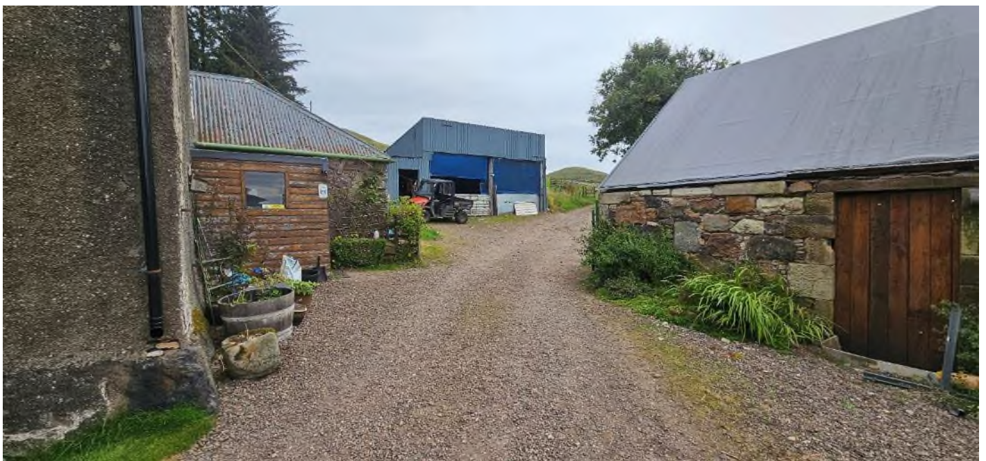
Figure 6: track leading north east with farmhouse on left and central steading to right. Hay barn beyond (Blue building).
