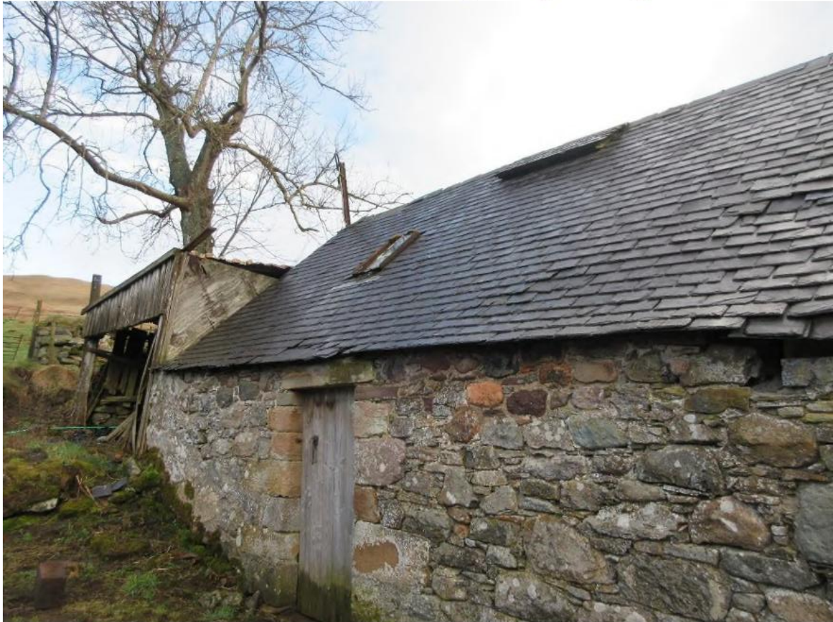
Photograph 4: showing a view of the external walls of the target building.
