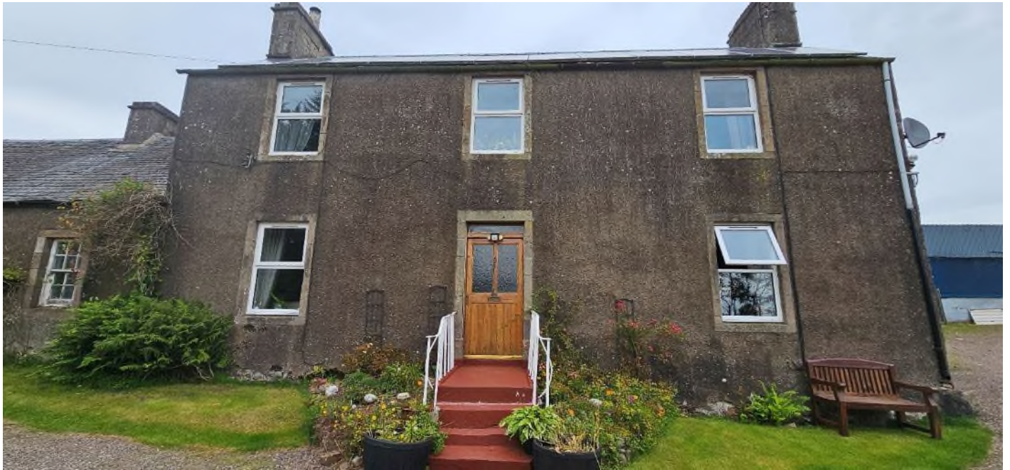
Figure 19: View of front of farmhouse. Note stepped access, harled with margins to windows and doors.
