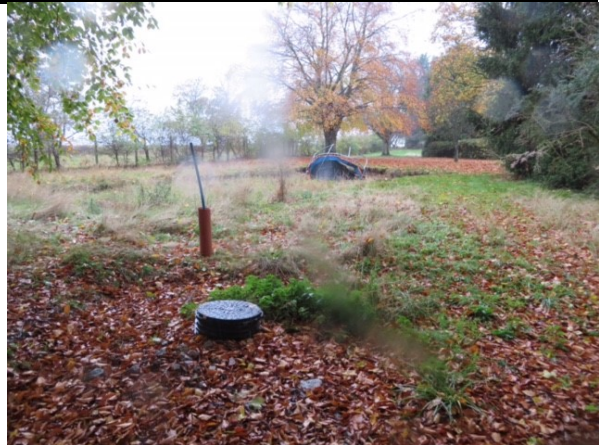
View towards SW, across application site, towards path running to the W of the site. (Excavated foundation of pool house and installed services in view).
