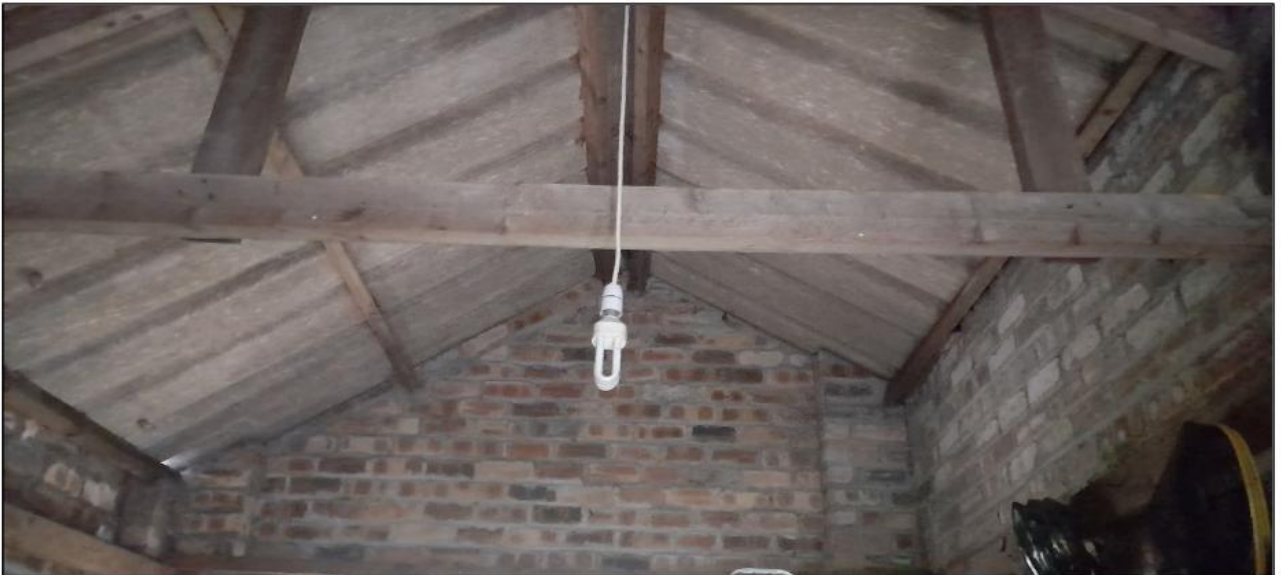
Photo 4: Inside the garage space
