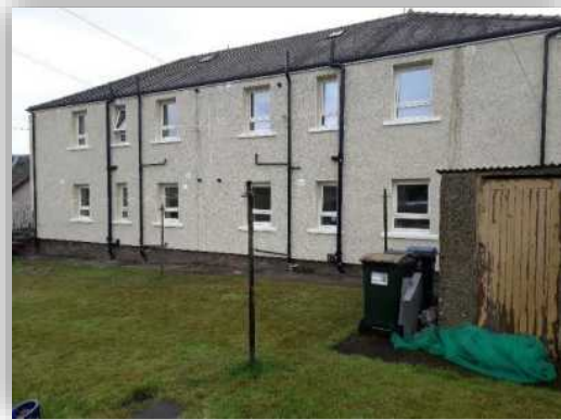
External Wall Insulation - High Street, Alyth
