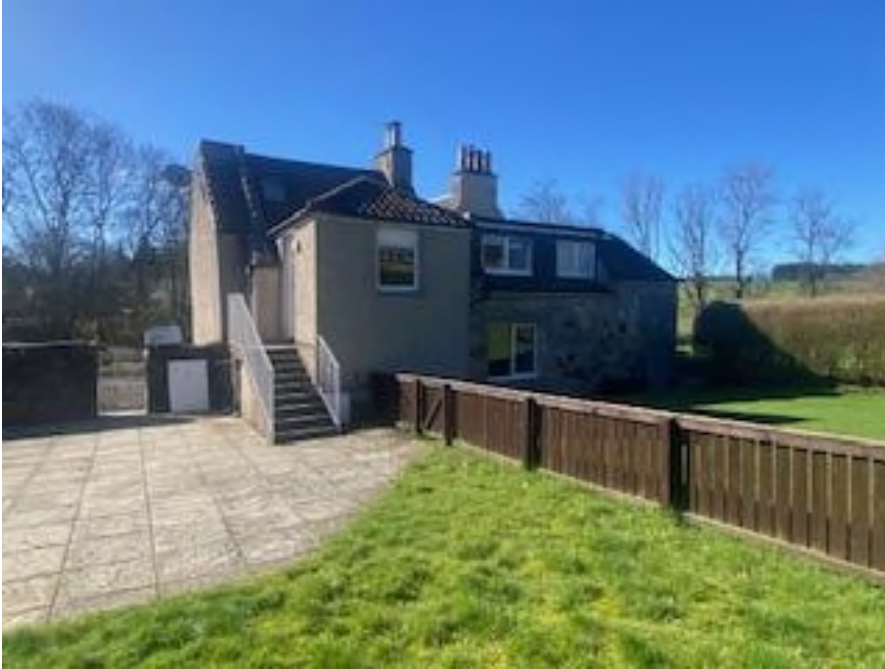
Photograph 9. Morning sunlight on northern elevation from existing two-storey host building.
