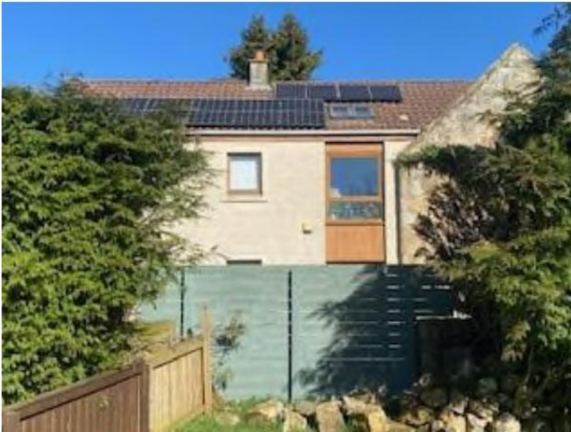
Photograph 8. Two storey projecting development off gable of house to north
