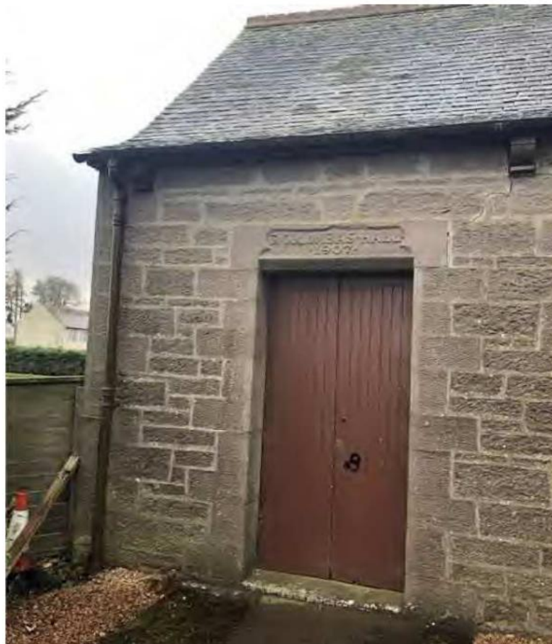
Figure 3.3: Church hall south-east entrance with 1907 date stone lintel
