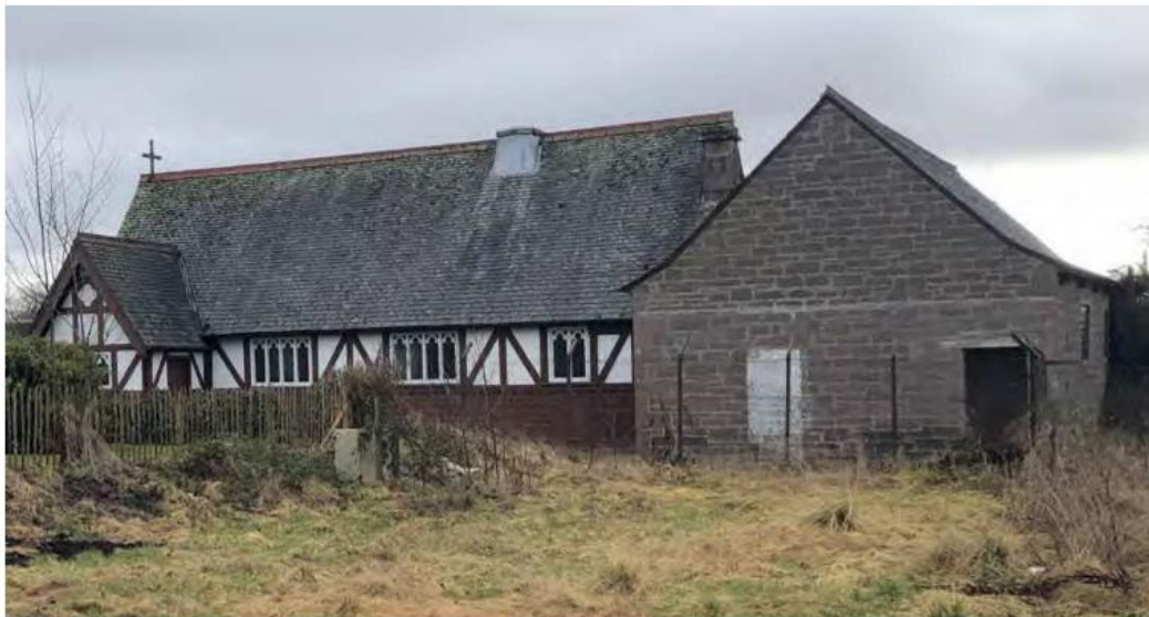
Figure 3.5: North elevations of St Columba's Episcopal Church (left) and church hall (right) showing the contrast in building materials, style and level of architectural detailing. The base for the now missing fleche on the church roof can be clearly seen in this image.
