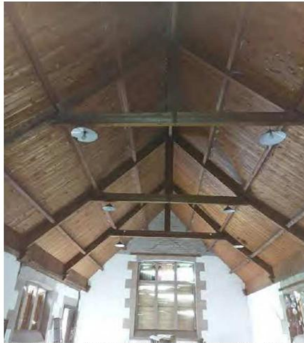
Figure 4: Site Photo Showing General Form of the Church Hall
