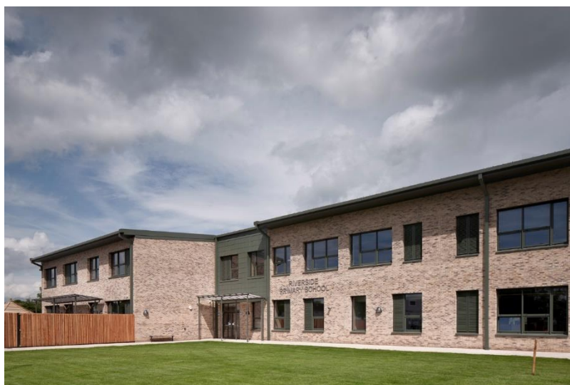
Riverside Primary School which opened in June 2023
