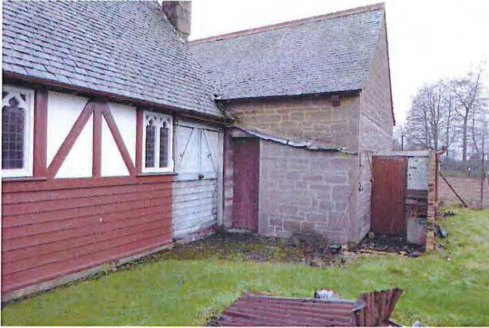
13 Partly demolished outbuildings, exposed/unpainted weatherboard.
