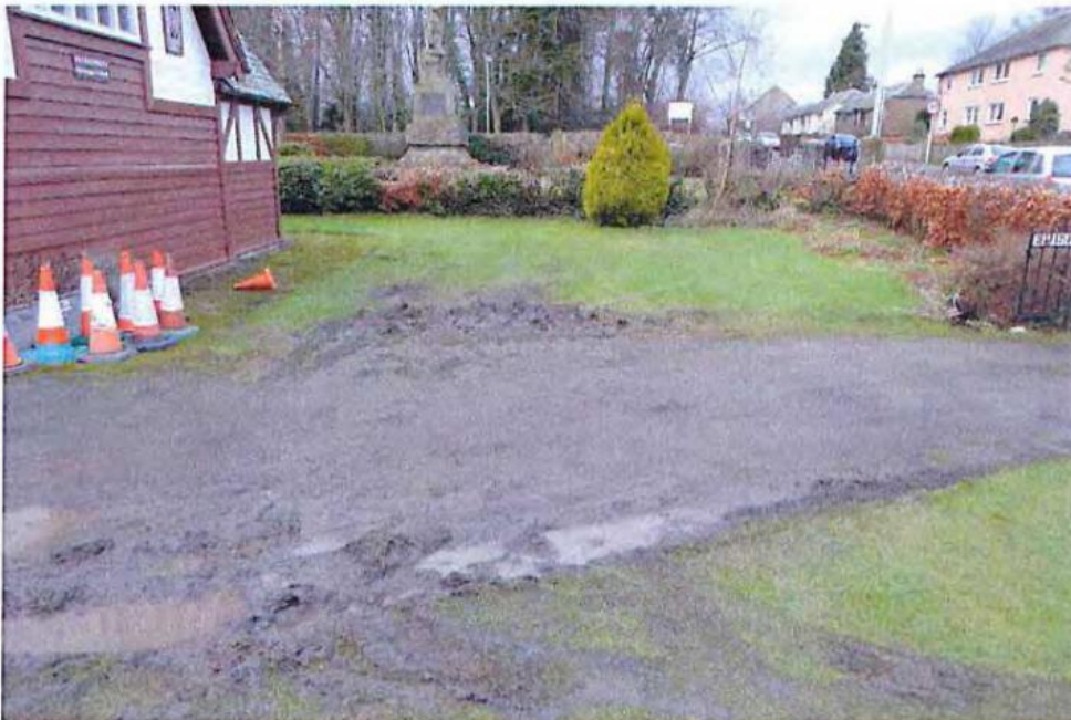
22 Access road/garden; moss on drive – no parking facilities, severe mud.
