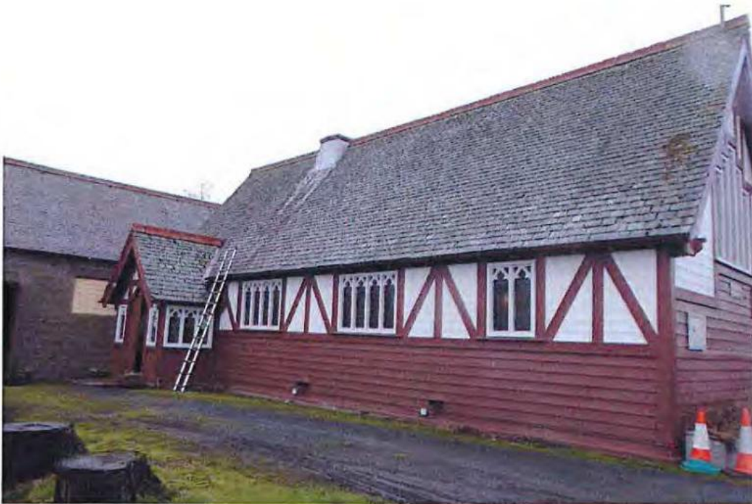
1 South elevation; shiplap weatherboarding to walls.
