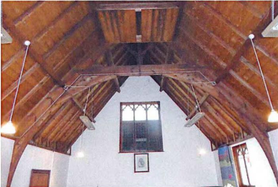
19 Church interior; timber trusses.
