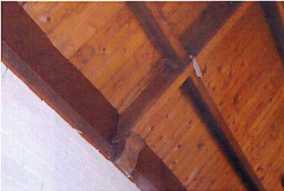
27 Truss supported on timber corbels.
