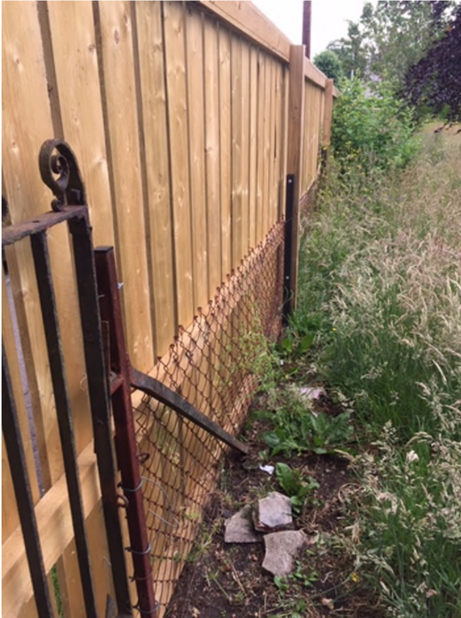
Photograph of new fence fixed to old fence
