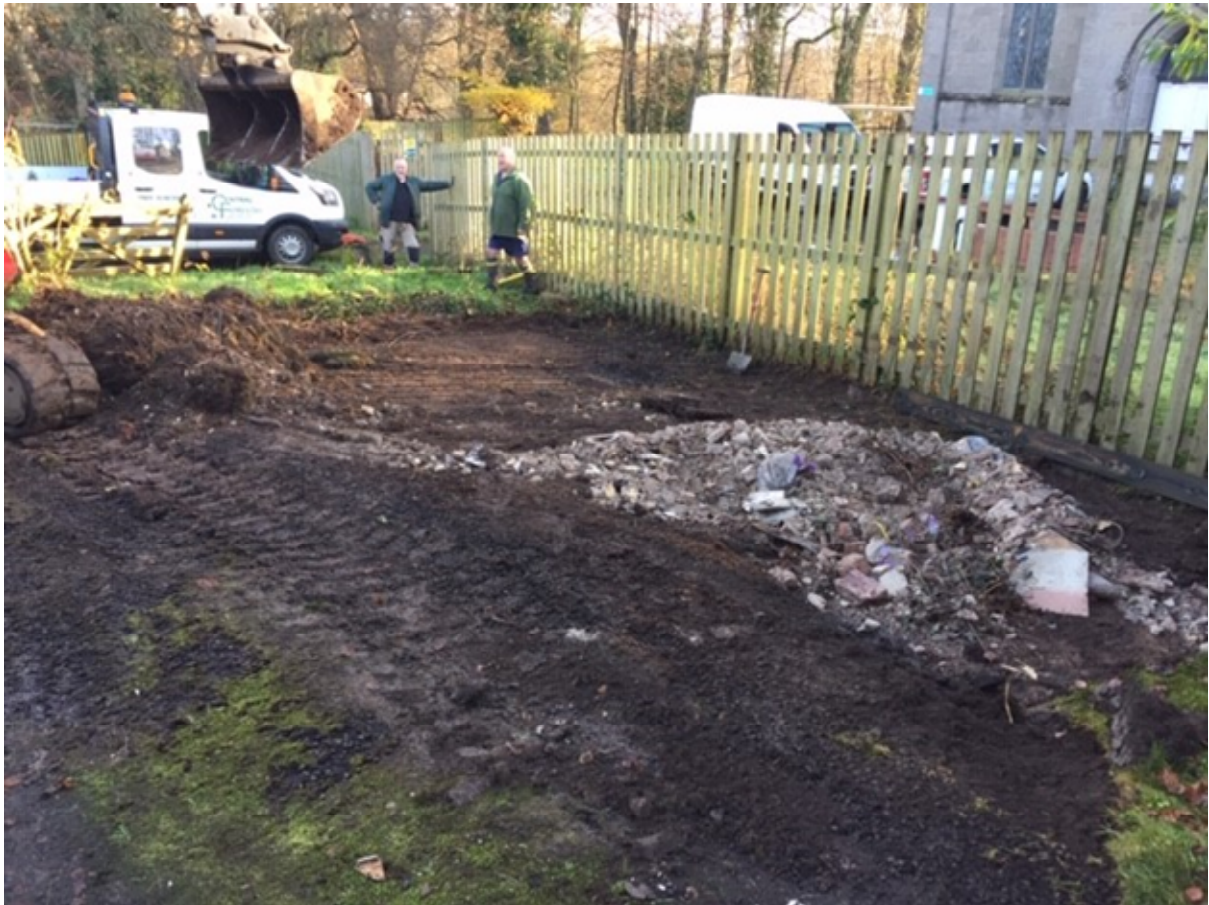
Photograph showing fence at other end of curtilage
