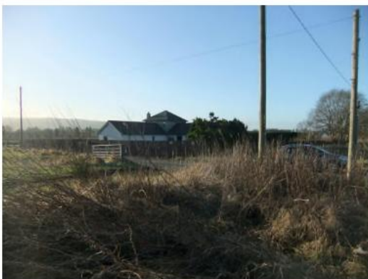
Uncharacteristic Turret roof extension
