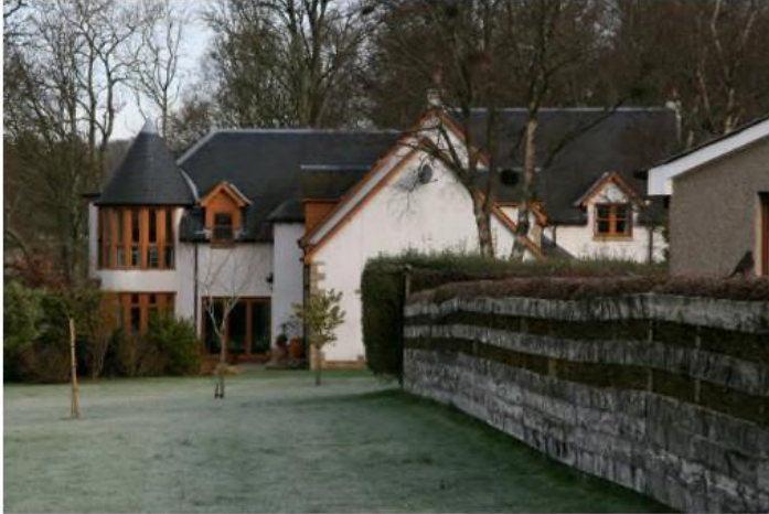
Darach Lodge (100m from application site) “uncharacteristic” Turret and Oriel Windows features?
