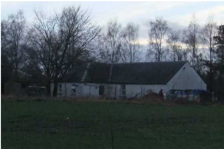
PRE-WAR SLATED ROOFS AT ROSEMOUNT
