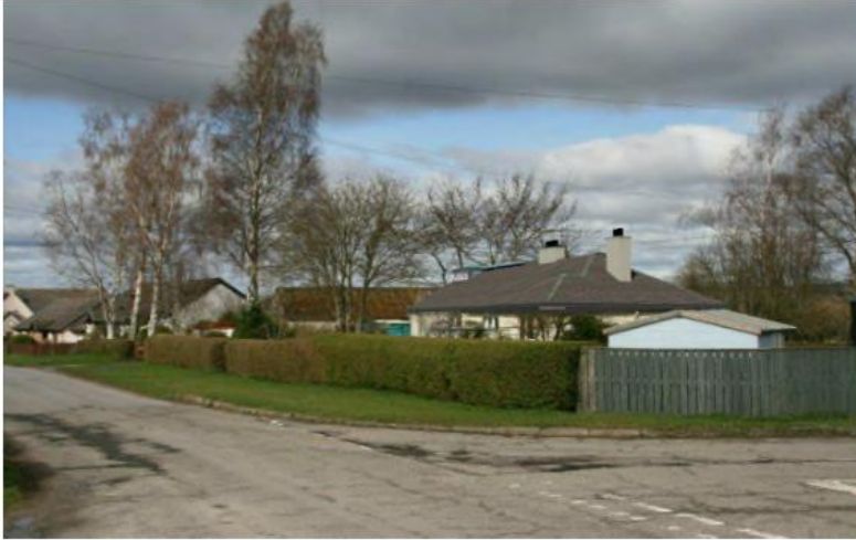
Application Site - Proposed roof extension viewed from the East
