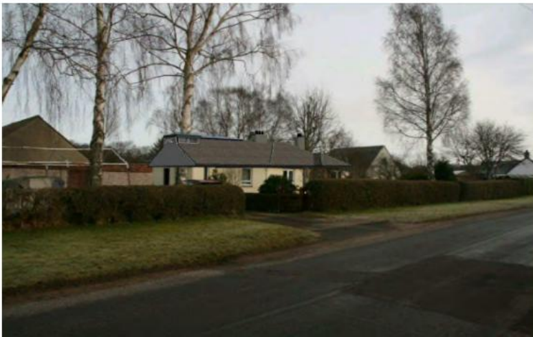
Proposed roof extension ridge shorter than neighbouring houses and gable end consistent with existing houses.
