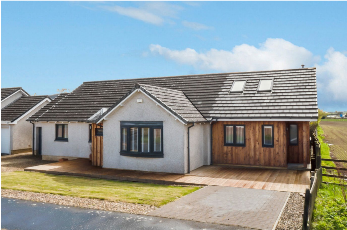
Figure 12 – Timber cladding used on extension to 21 Hatchbank Road
