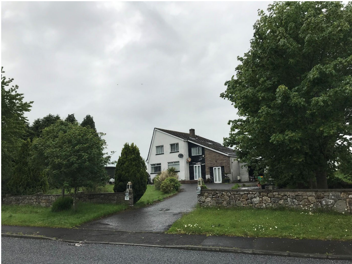
Figure 11 – View of house showing containment/ screening to the South-West corner of the site along with containment to the East and black timber existing to the house
