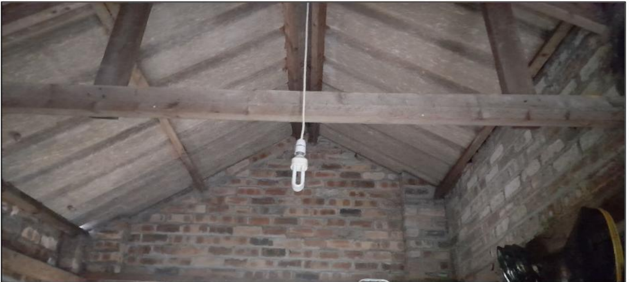
Photo 4: Inside the garage space
