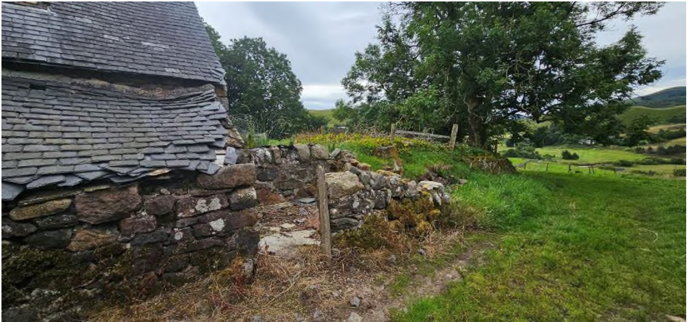
Figure 9: Location of former shed to south of steading.
