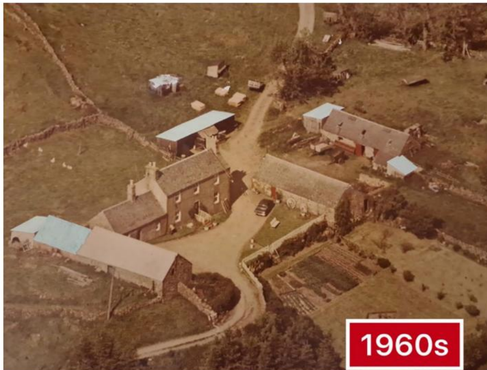
Figure 6: Former lean-to located to north and south of steadings. Shown by tin roof
