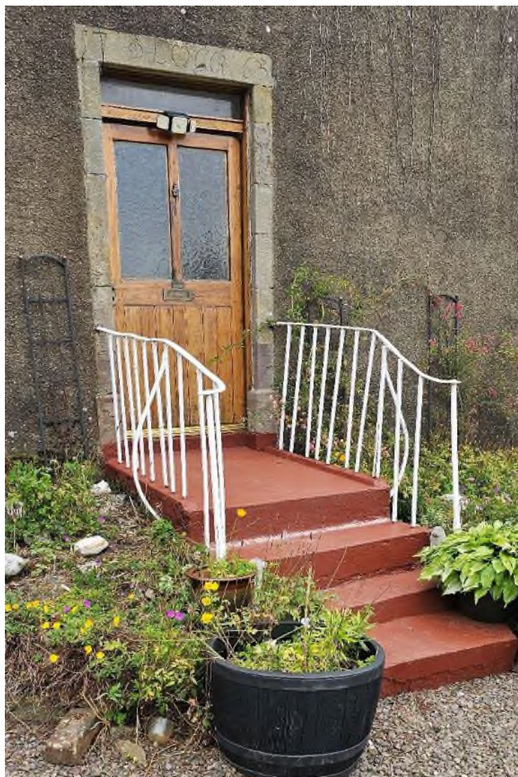
Figure 20: Closer view of front door with stepped access
