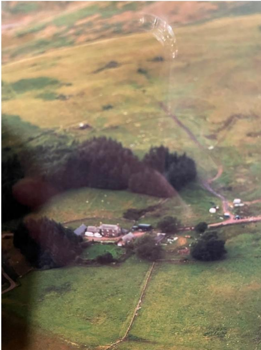
Figure 1: image from 1980's showing form of buildings on the site. The extensions to north, south and east of the steading subject to this application can be seen
