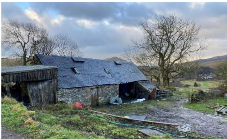
Figure 2: View of steading subject of this appraisal
