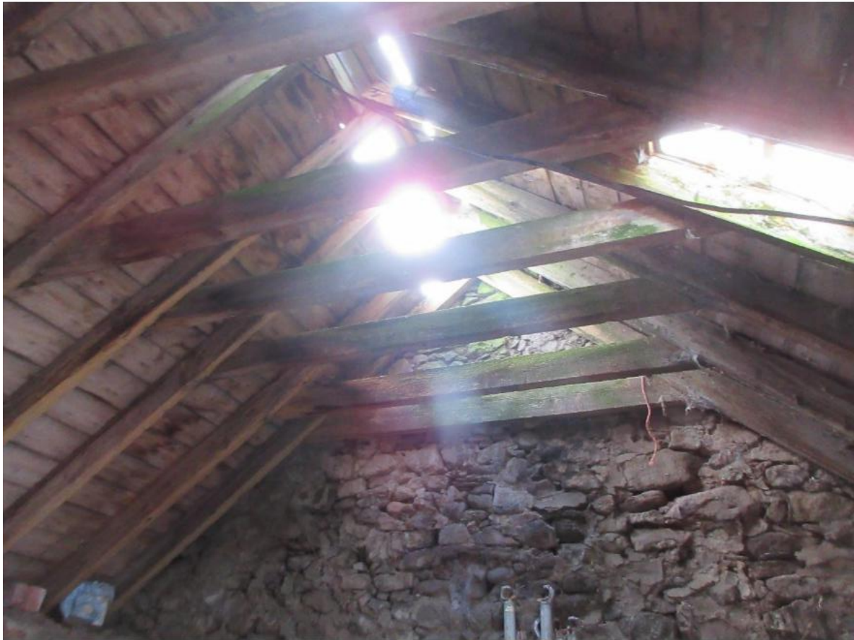
Photograph 5: showing a view of the ridge of the building
