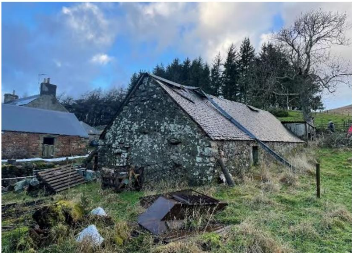
Figure 8: Picture of the steading showing current disrepair
