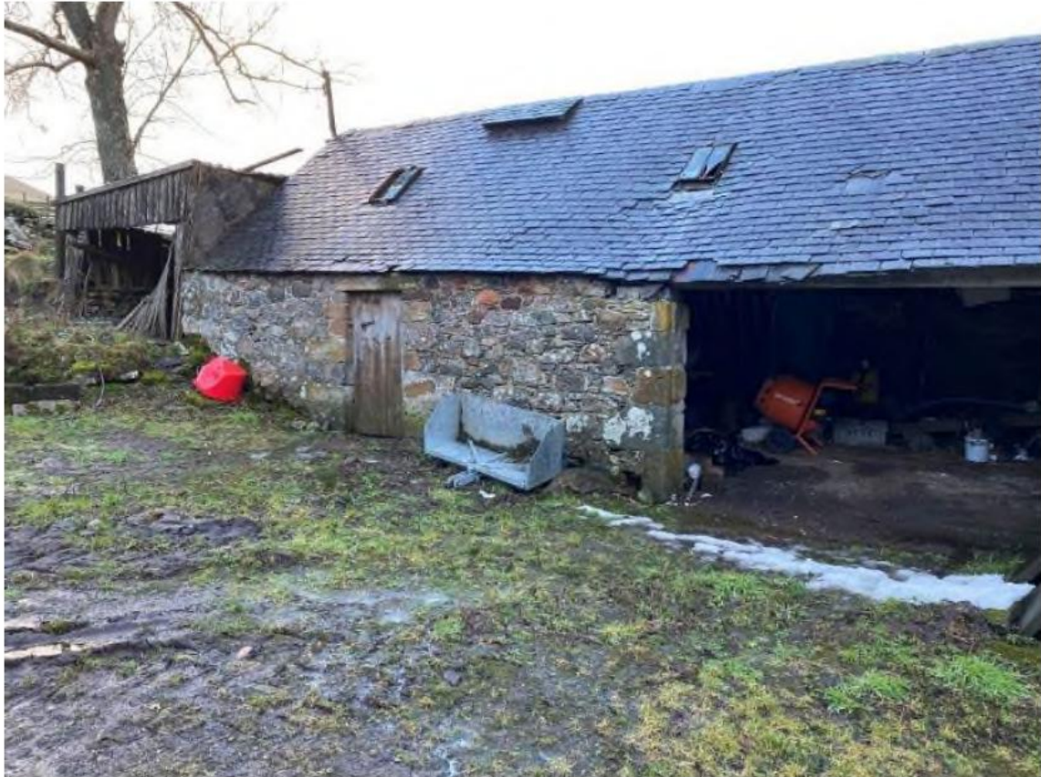
Figure 9: Picture of the steading showing current disrepair
