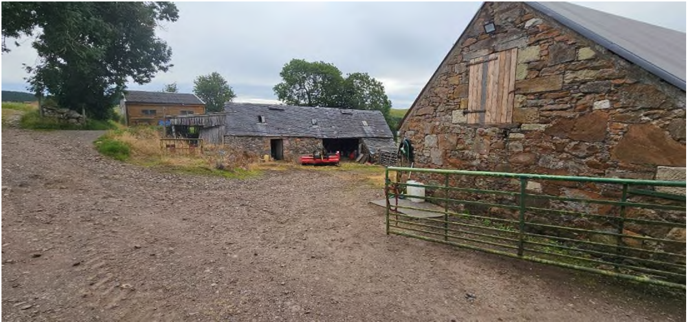
Figure 7: First view of steading subject to proposals. Stable beyond to the east.
