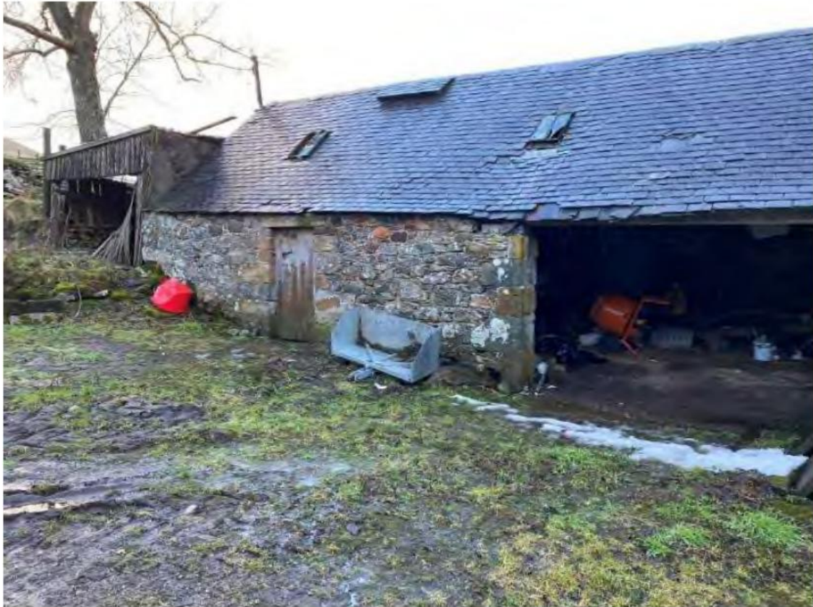
Figure 8: Picture of the steading showing current disrepair
