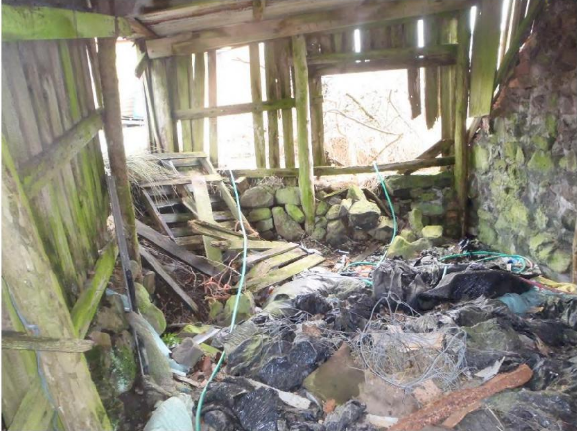
Photograph 6: showing a view of the lean-to structure located north of the main building
