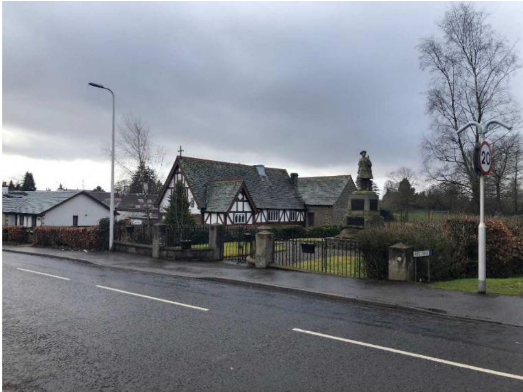
Figure 3.6: View from Perth Road, looking south-east and showing the spatial relationship between St Columba’s Episcopal Church and the war memorial, which are situated within adjacent, but separate plots. Modern single storey residential buildings are visible beyond the church detracting from its intended local prominence.
