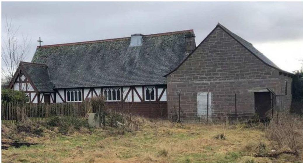
Figure 3.5: North elevations of St Columba's Episcopal Church (left) and church hall (right) showing the contrast in building materials, style and level of architectural detailing. The base for the now missing fleche on the church roof can be clearly seen in this image.
