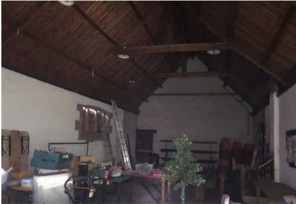
Figure 3.4: Church hall interior, currently disused
