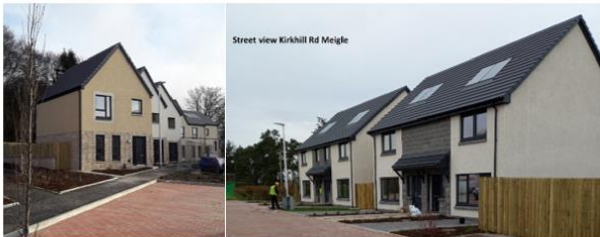
New Build Housing in Scone and Meigle
