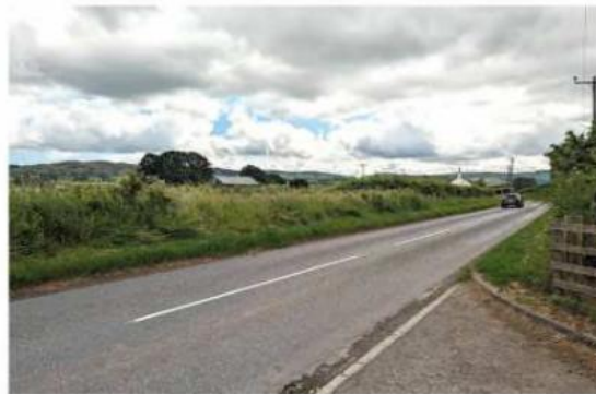
Image showing view from Drumearn Junction July 23
