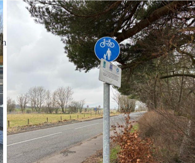
Shared-use facility- Cleish to Crook of Devon
