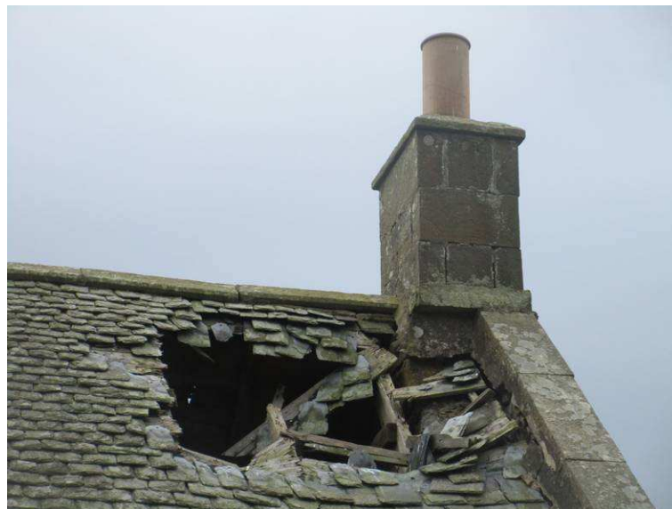
Fig. 15: North elevation showing hole in roof.
