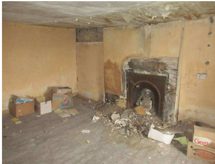
Fig. 19: Interior showing fireplace 2 and deteriorating linings.
