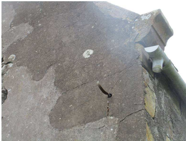
Fig. 12: Missing rainwater goods, original bracket.
