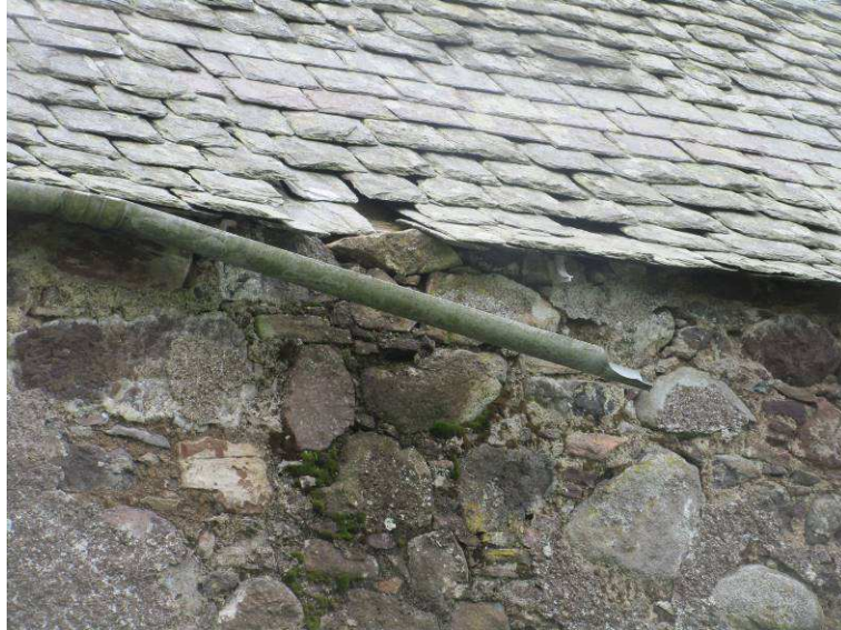
Fig. 11: Broken & Missing PVC rainwater goods.
