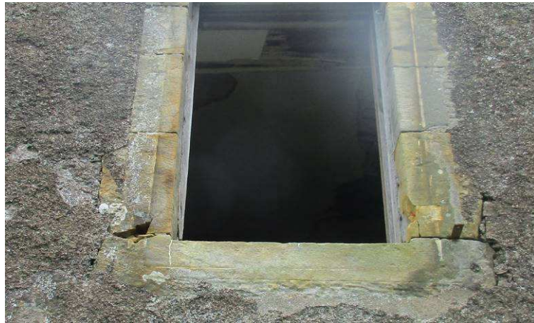
Fig. 8: Damaged stonework from shutter fixings
