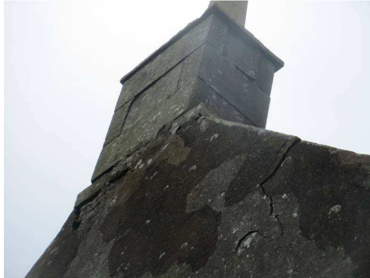
Fig. 9: Loose stones in chimney.
