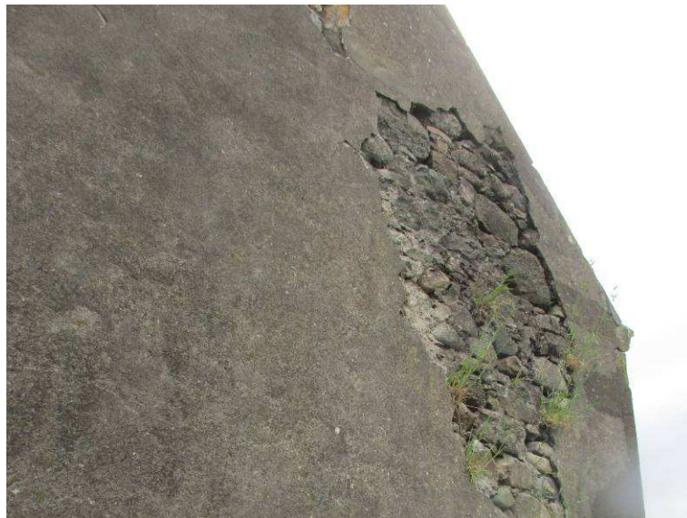
Fig. 6: Failing render and vegetation.
