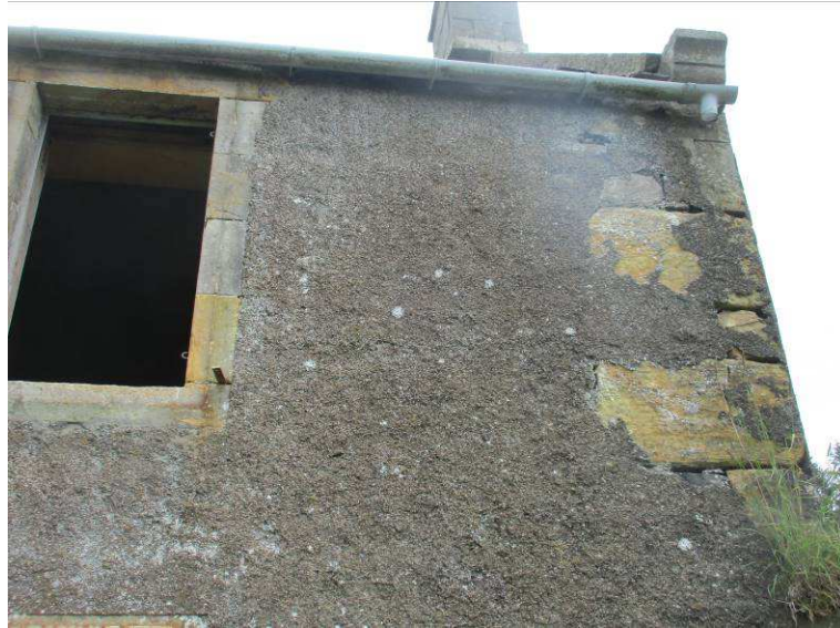
Fig. 7: Lime harling on south facade
