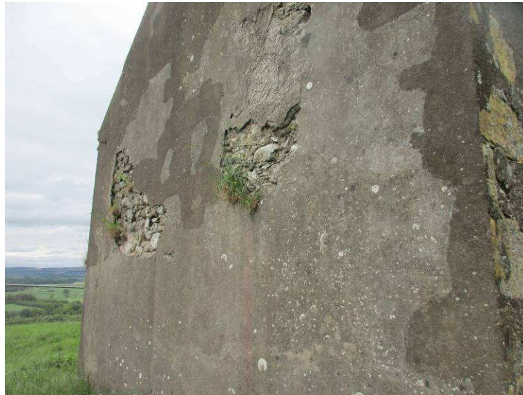
Fig. 5: Gable Elevation with cement render failure.
