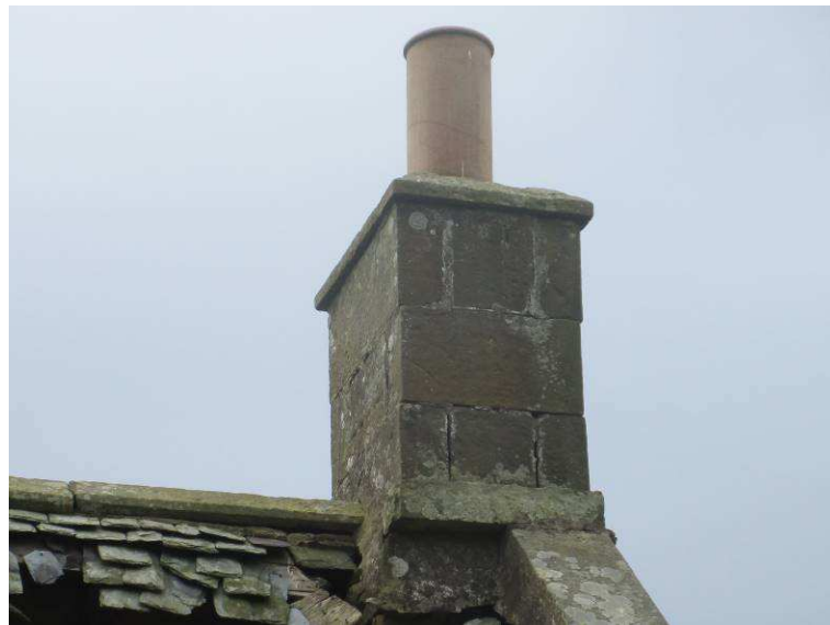
Fig. 10: Chimney to be repointed.
