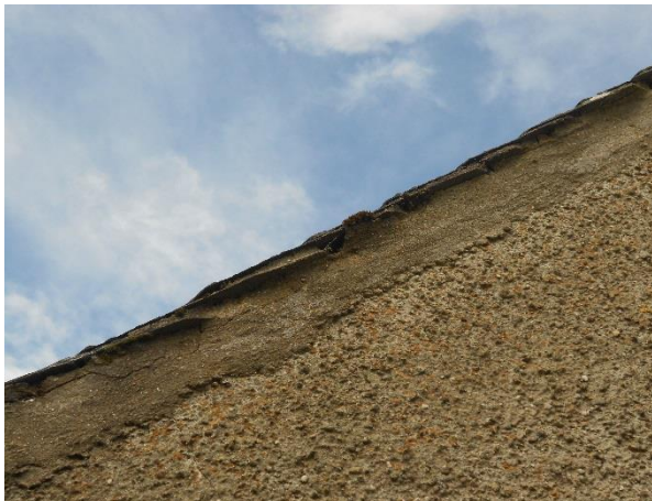
Photograph 8: Gap in mortar on gable end on south elevation
