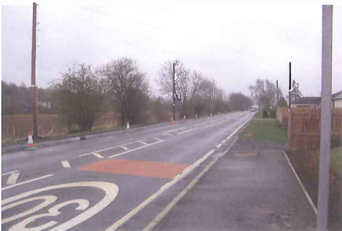
Photograph 2 – A view looking south along the B867 from the frontage of “Hillview”. The new footway on the eastern side of the road can be seen with new offlets incorporated.
