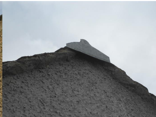
Photograph 9: Gap behind zinc ridge end cap on north elevation
