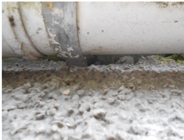
Photograph 12: Gaps visible under zinc ridge.
