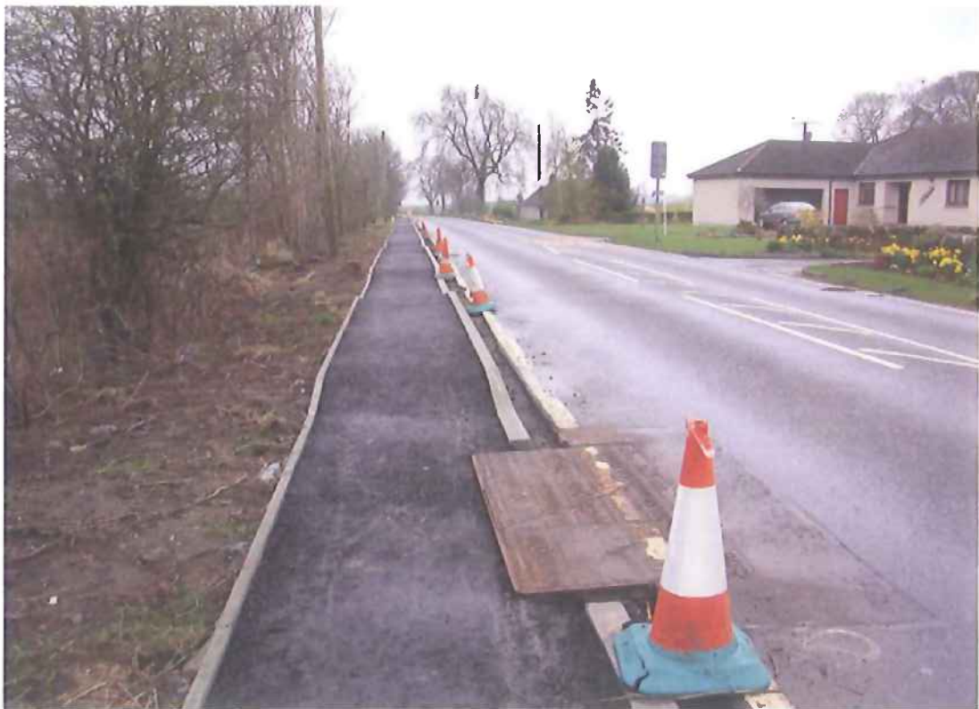
Photograph 4 – Looking southwards along the B867. The offlets constructed in the new footway are clearly seen in this picture.
