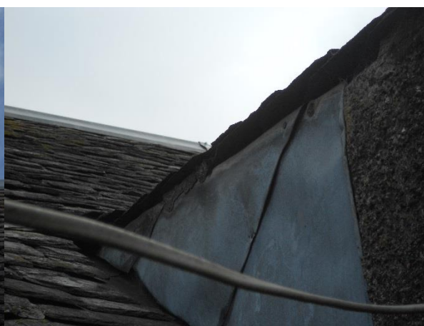
Photograph 13: Gaps between the lead flashing and slates tying in the lean-to.
