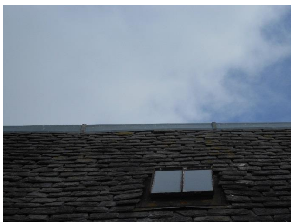
Photograph 12: Gaps visible under zinc ridge.
