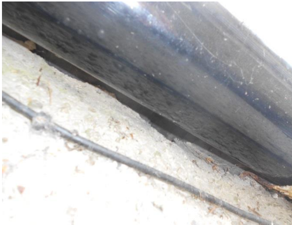
Photograph 8: Gap in mortar on gable end on south elevation
