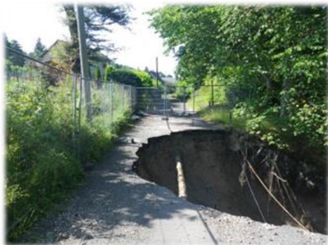
Figure 11. Landslide caused by flooding above
