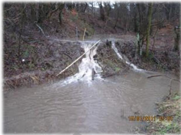
Figure? Pipe became blocked during heavy rainfall contributing to flooding within a housing estate and a main access road.
