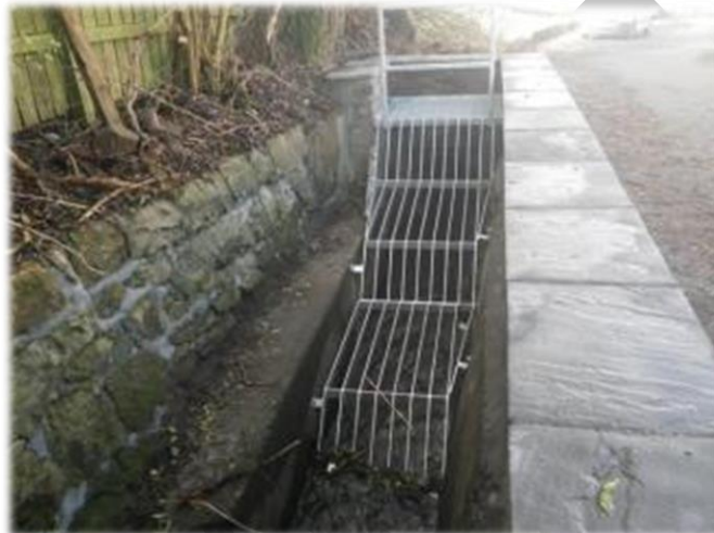
Figure? New trash screen installed along with major pipe upgrade to alleviate flooding
