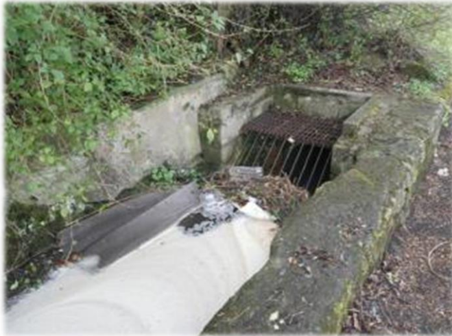
Figure? Key flood locations trash screen in Cambusbarron prior to upgrade
