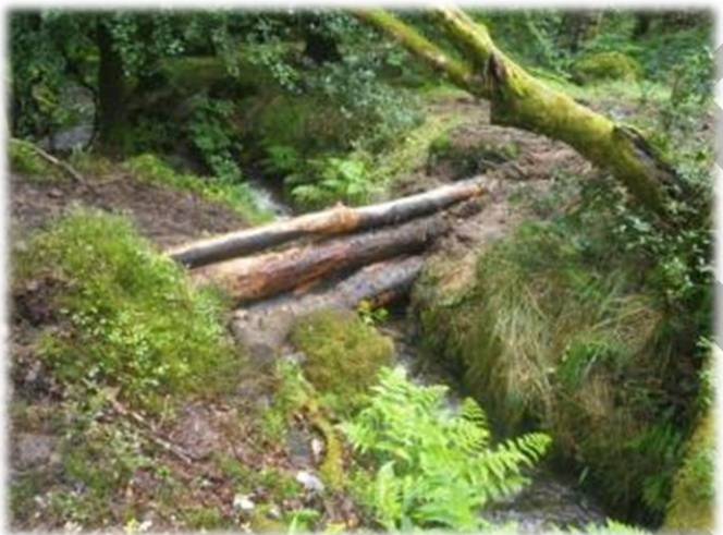
Figure 7: Leaky dams on one of the watercourses running from the Craggs in Callander
