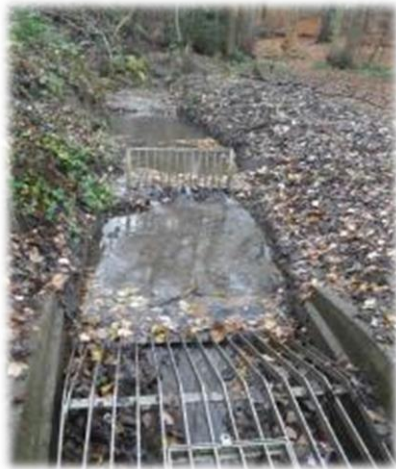
Figure? Trash screen and pipe inlet before upgrade
