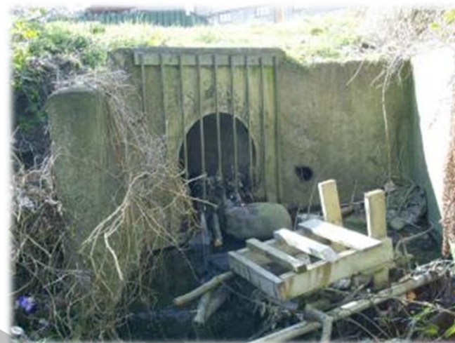
Figure? Fly-tipped debris built up at outfall prevents gulleys emptying into the pipes .Results in flooding on roads and footpaths
