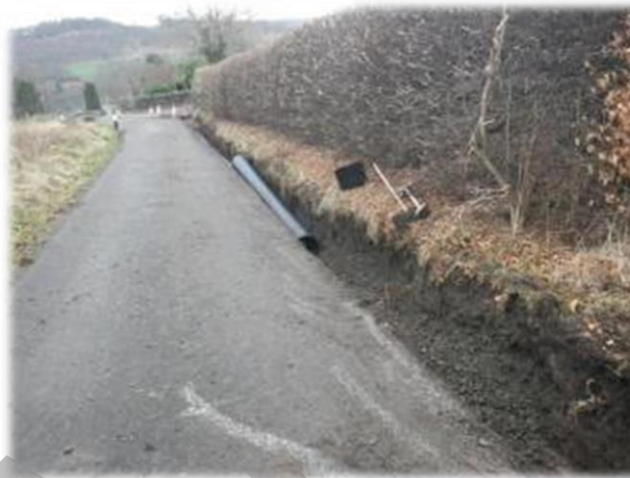
Figure 13: Maintenance. Extensive new roadside drainage installed to alleviate surface water flooding
