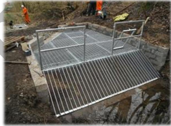
Figure? New trash screen installed and maintained by the council fortnightly. No reported flooding since installation completed.
