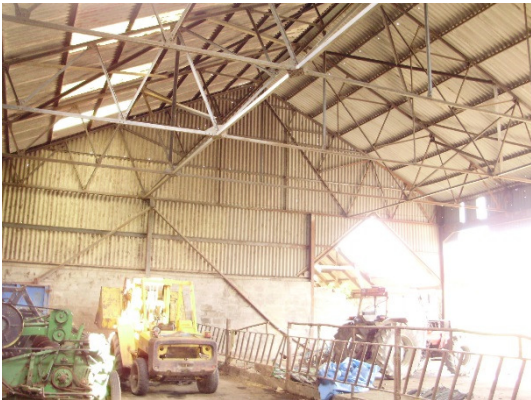
Photograph 15: Gaps between flashing and roof sheeting in Building 5
