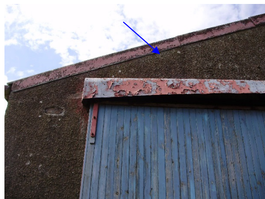
Photograph 10: Crack in brickwork and gap under barge board in Building 1
