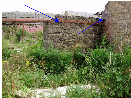
Photograph 16: Gaps in stonework in Building 5
