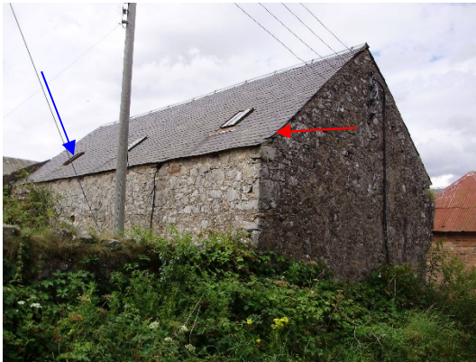
Photograph 21: Gaps under missing slates and metal flashing in Building 9
