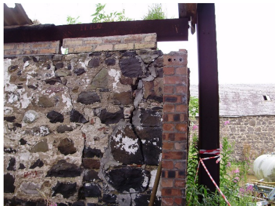
Photograph 16: Gaps in stonework in Building 5
