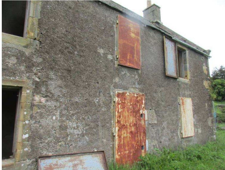
Fig. 13: Protective metal shuttering to south facade
