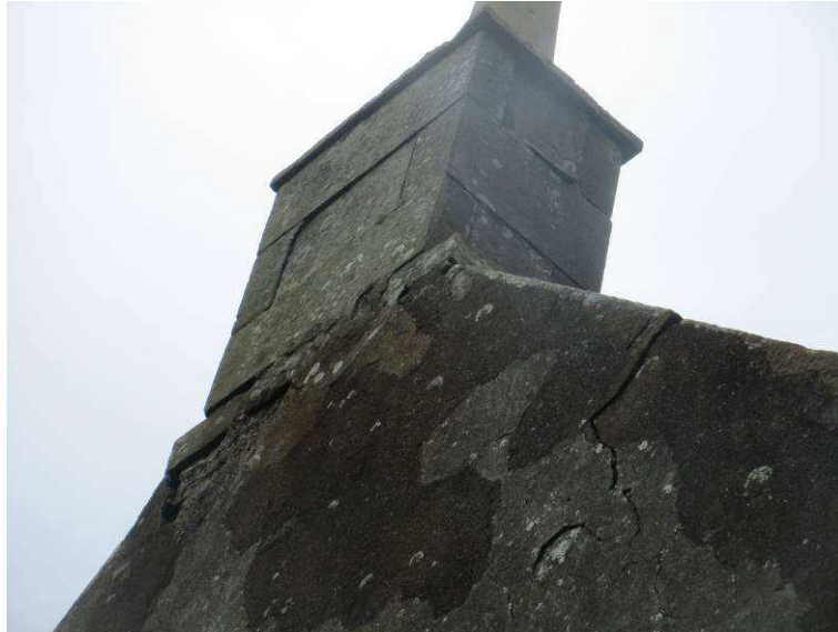
Fig. 9: Loose stones in chimney.
