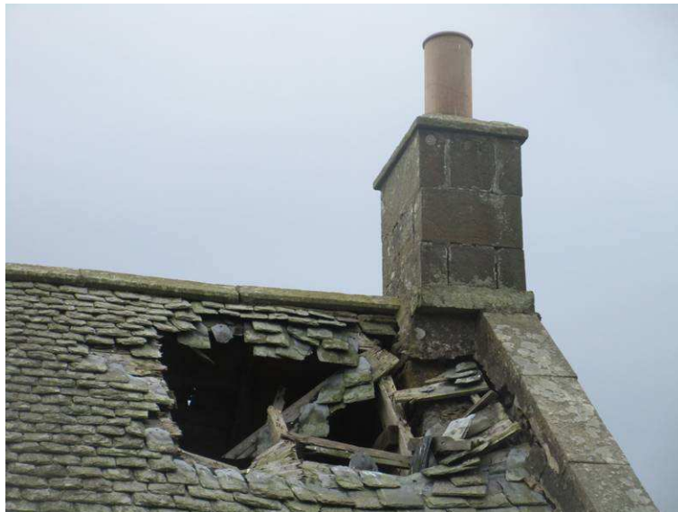
Fig. 15: North elevation showing hole in roof.
