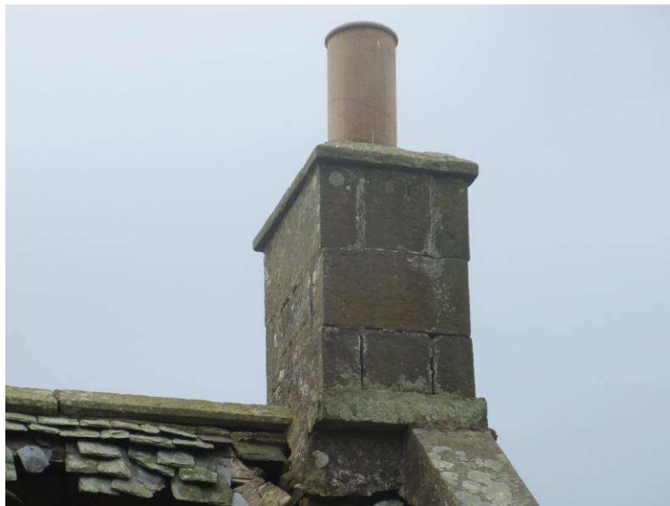
Fig. 10: Chimney to be repointed.
