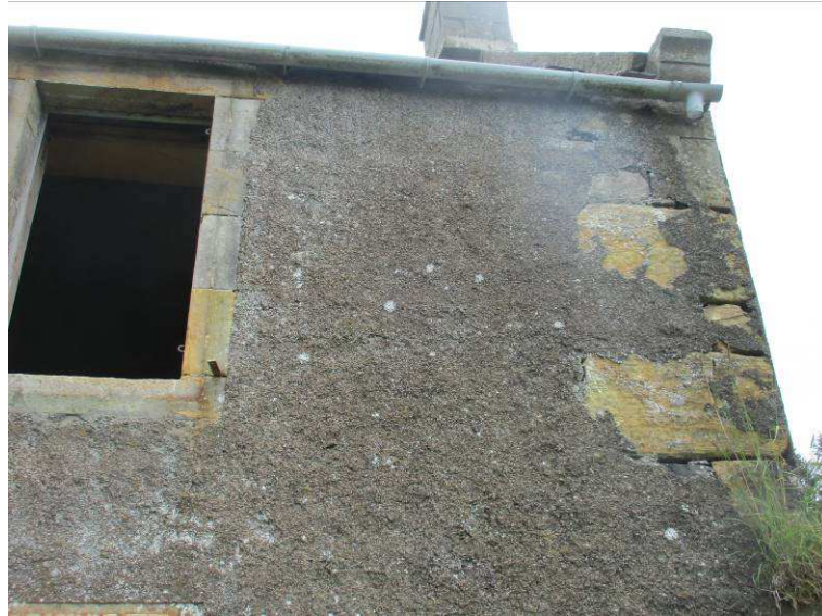
Fig. 7: Lime harling on south facade
