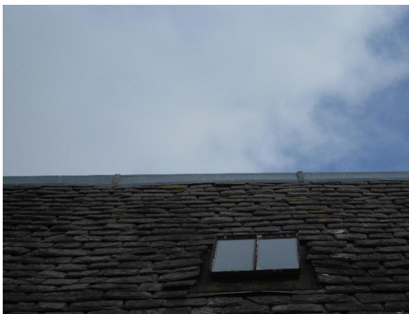
Photograph 12: Gaps visible under zinc ridge.
