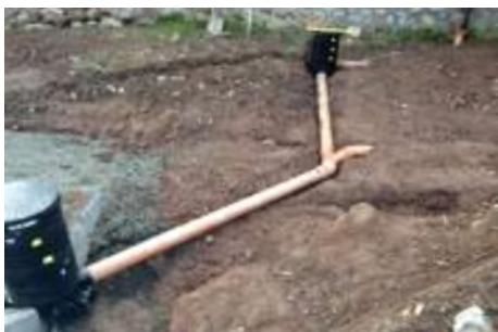
Pipework & Inspection Chamber
