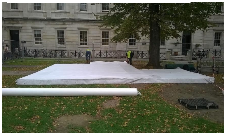
Section Of Arbor Raft Complete With Geotextile
