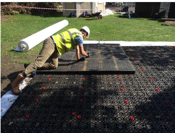
Installing Arbor Raft Two Units High
