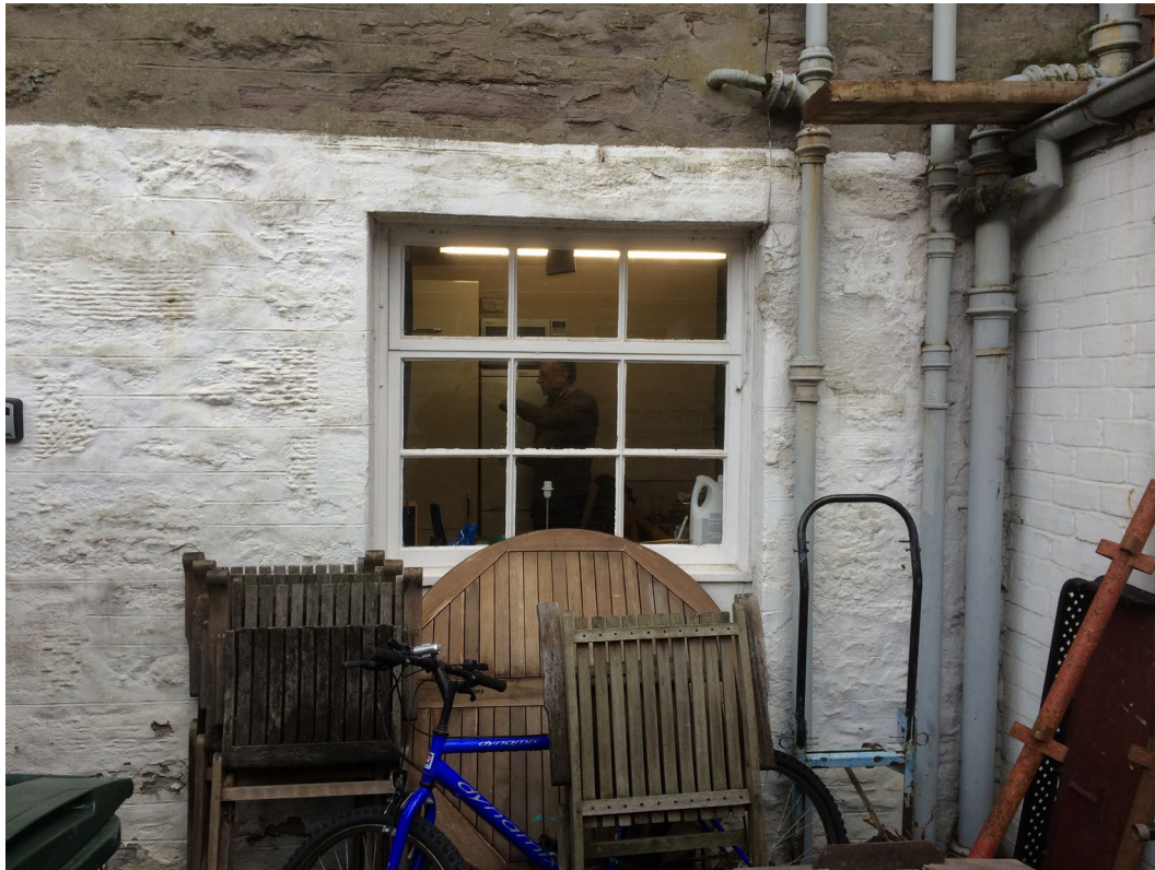
Existing Window W1 – Painted Timber Casement Window with Astragals – Top hung hopper. – To be removed.
