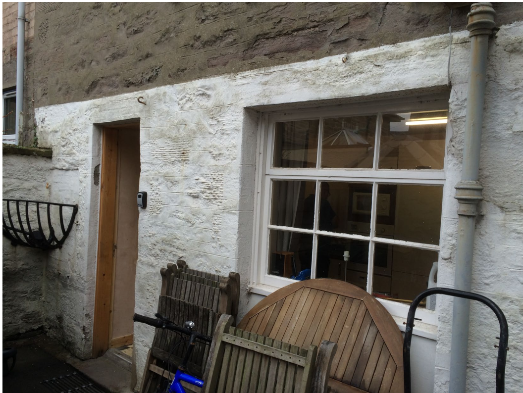
Existing Window W1 – Painted Timber Casement Window with Astragals & Top hung hopper. – Remove Window, Cill & Underbuild, Retain Structural Opening. Fit new UPVC Double Glazed Patio Door with astragals.
