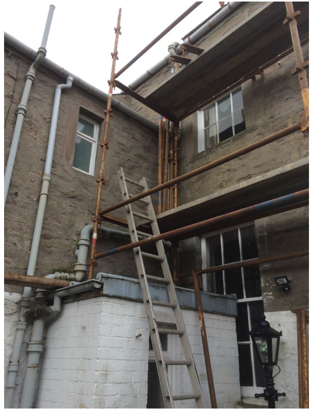
1.0 - View from rear courtyard prior to alterations - Flat Roofed White Painted Brick WC structure to be removed. Note how this structure abuts directly the existing sliding sash window of the main two storey dwelling.
