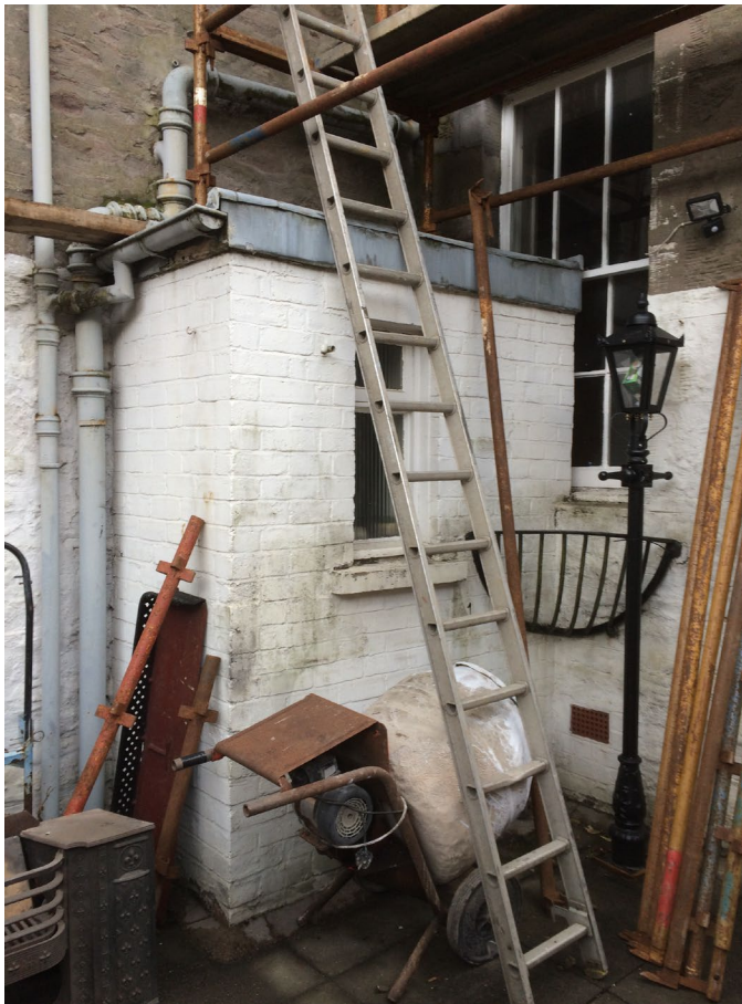
Existing Flat Roofed Painted Brick WC structure to be removed.
