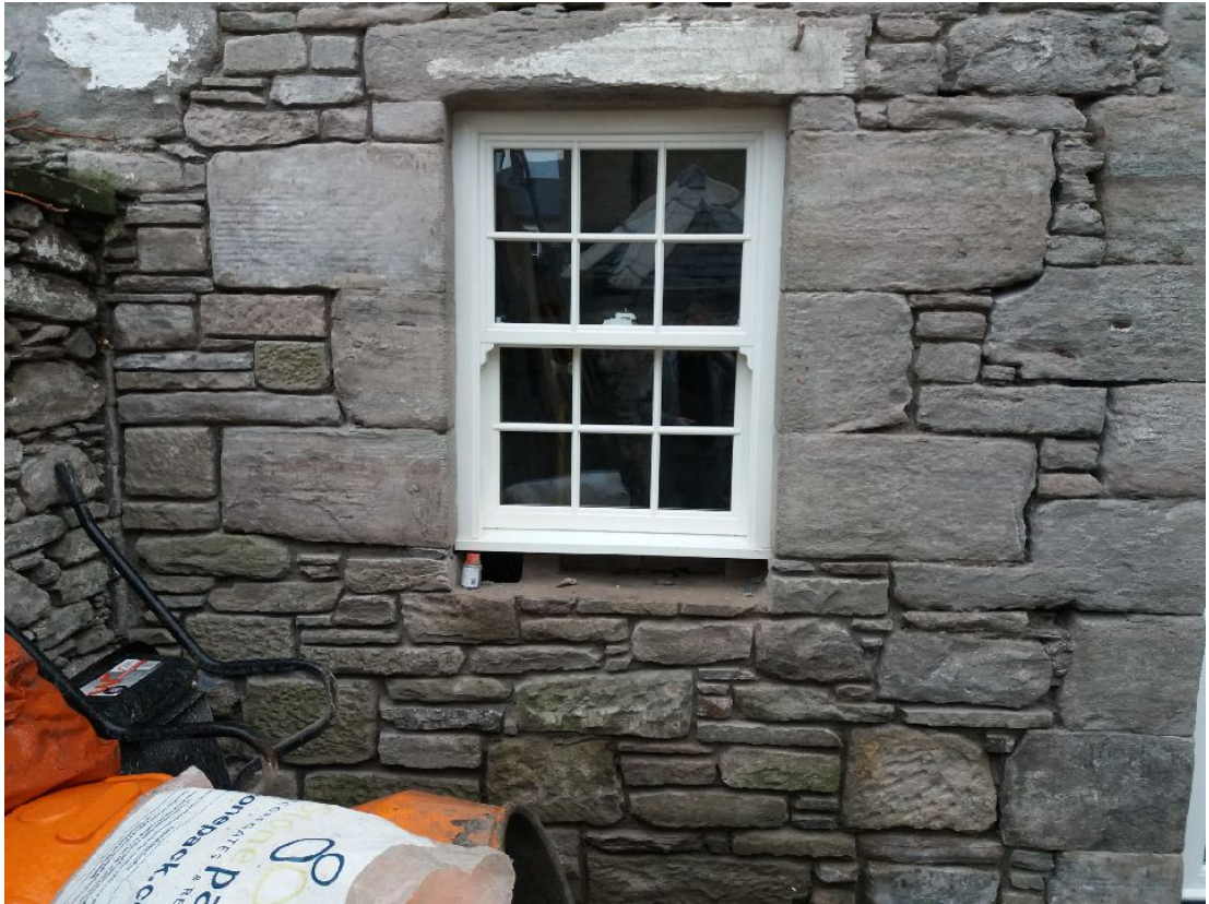
New W3 Fitted – White UPVC Double Glazed Sliding Sash Windows with Astragals.
