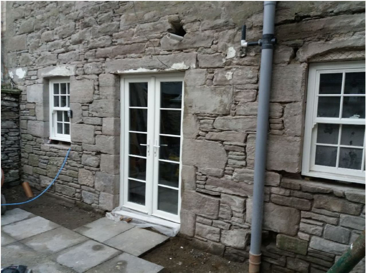
New Fitted W4, D2 & W3. White Upvc framed double glazed Sliding Sash Windows & White Upvc framed Patio Door with Astragals - Whitewash removed & stone finish restored.
