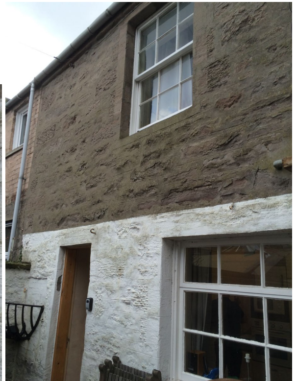
2.0 - View from rear courtyard prior to alterations - White Painted ground floor stonework with existing door and top hinged casement window.
