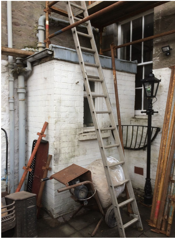
1.0 - View from rear courtyard prior to alterations - Flat Roofed White Painted Brick WC structure to be removed. Note how this structure abuts directly the existing sliding sash window of the main two storey dwelling.
