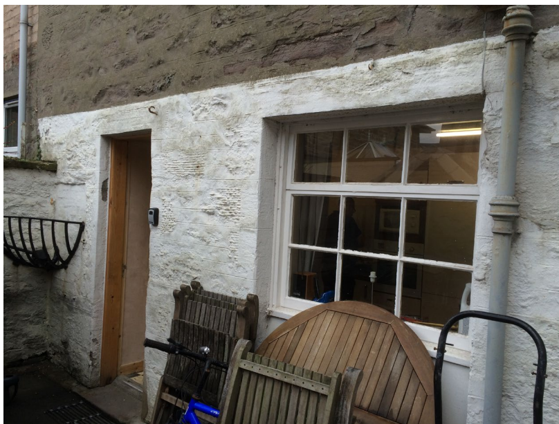
2.0 - View from rear courtyard prior to alterations - White Painted ground floor stonework with existing door and top hinged casement window.
