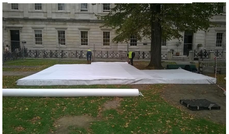
Section Of Arbor Raft Complete With Geotextile
