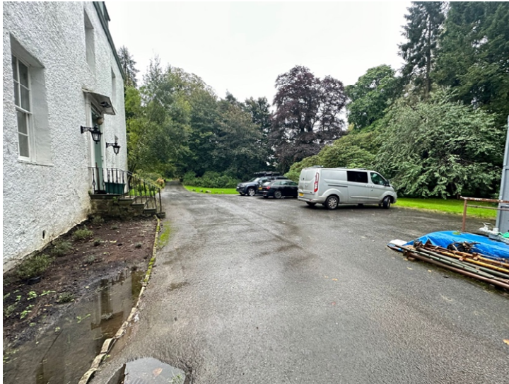
The front of the house and puddle, this was due to the drain you can see in bottom left which had become blocked, it has since been cleared and such puddling has not happened again.
