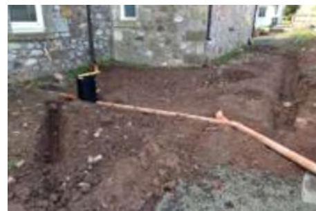
Pipework & Inspection Chamber
