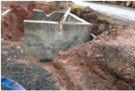
Concrete Bund to Protect Treatment Plant
