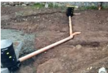
Pipework & Inspection Chamber
