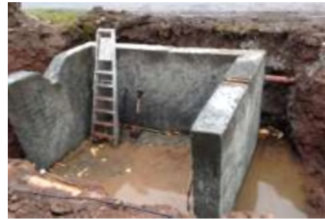
Concrete Bund to Protect Treatment Plant
