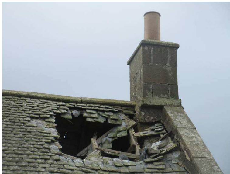
Fig. 15: North elevation showing hole in roof.
