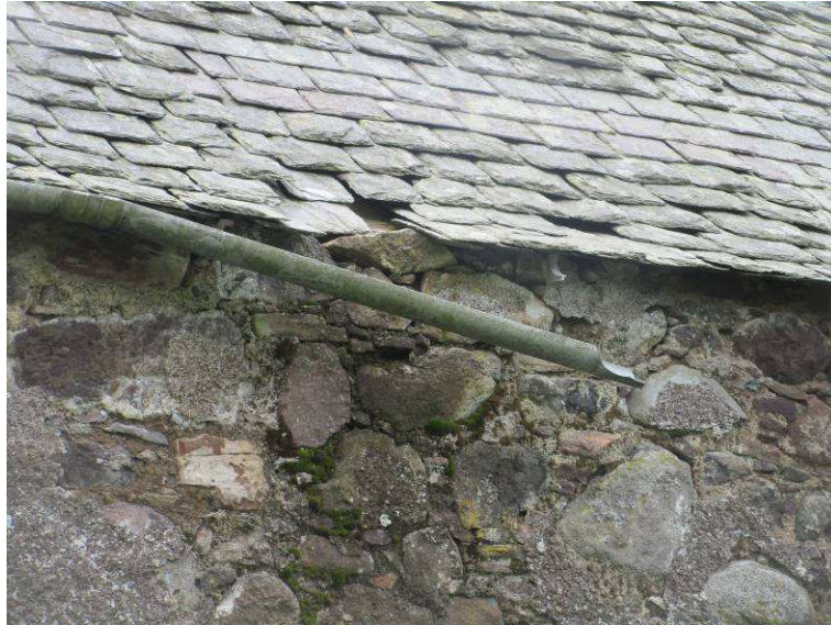
Fig. 11: Broken & Missing PVC rainwater goods.
