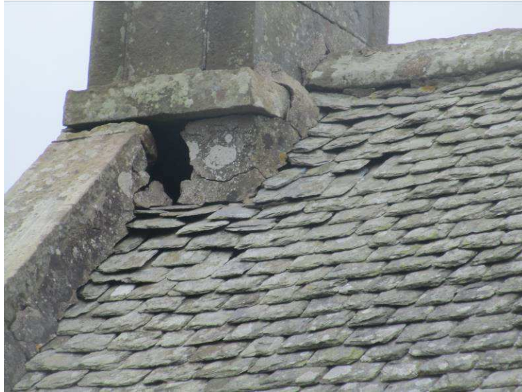
Fig. 16: North elevation showing hole in roof.
