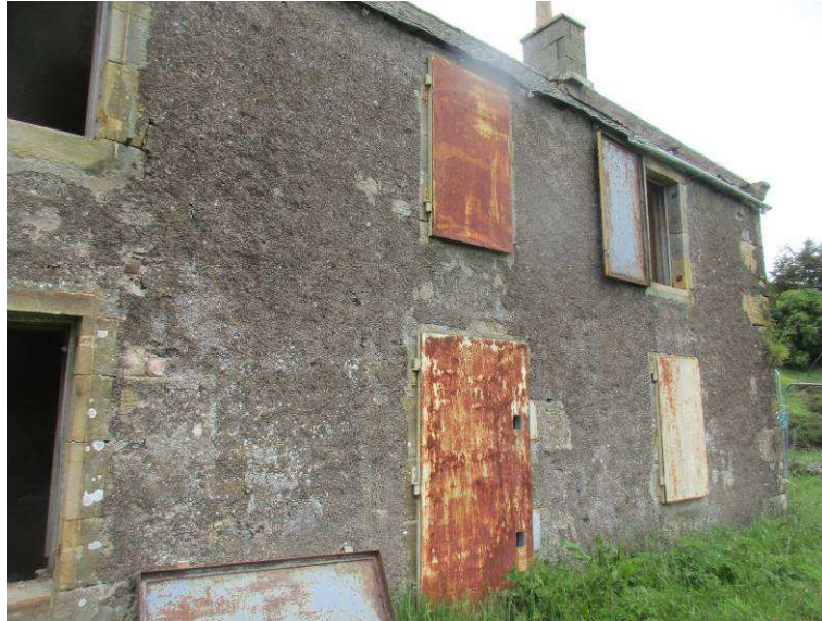
Fig. 13: Protective metal shuttering to south facade
