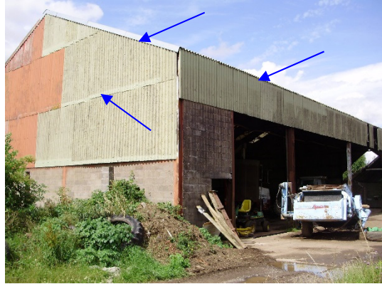
Photograph 14: Gaps in stonework, under flashing and between steelwork in derelict Building 4
