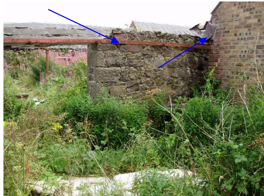
Photograph 16: Gaps in stonework in Building 5
