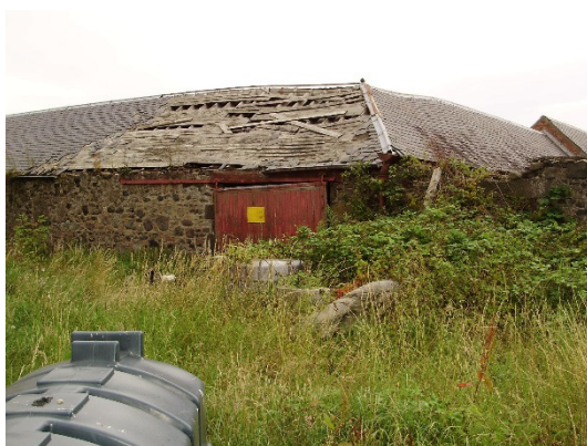
Photograph 21: Gaps under missing slates and metal flashing in Building 9
