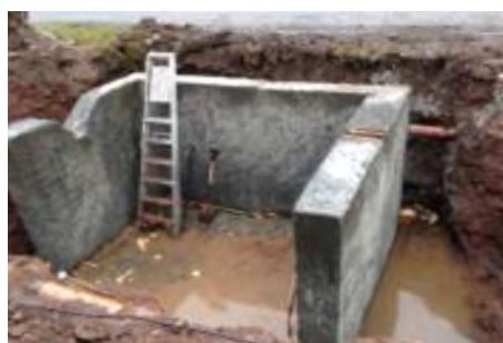
Concrete Bund to Protect Treatment Plant
