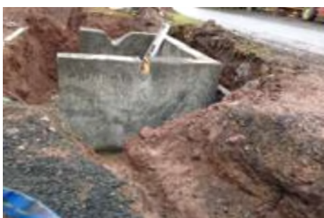
Concrete Bund to Protect Treatment Plant
