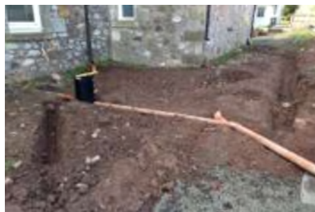
Pipework & Inspection Chamber
